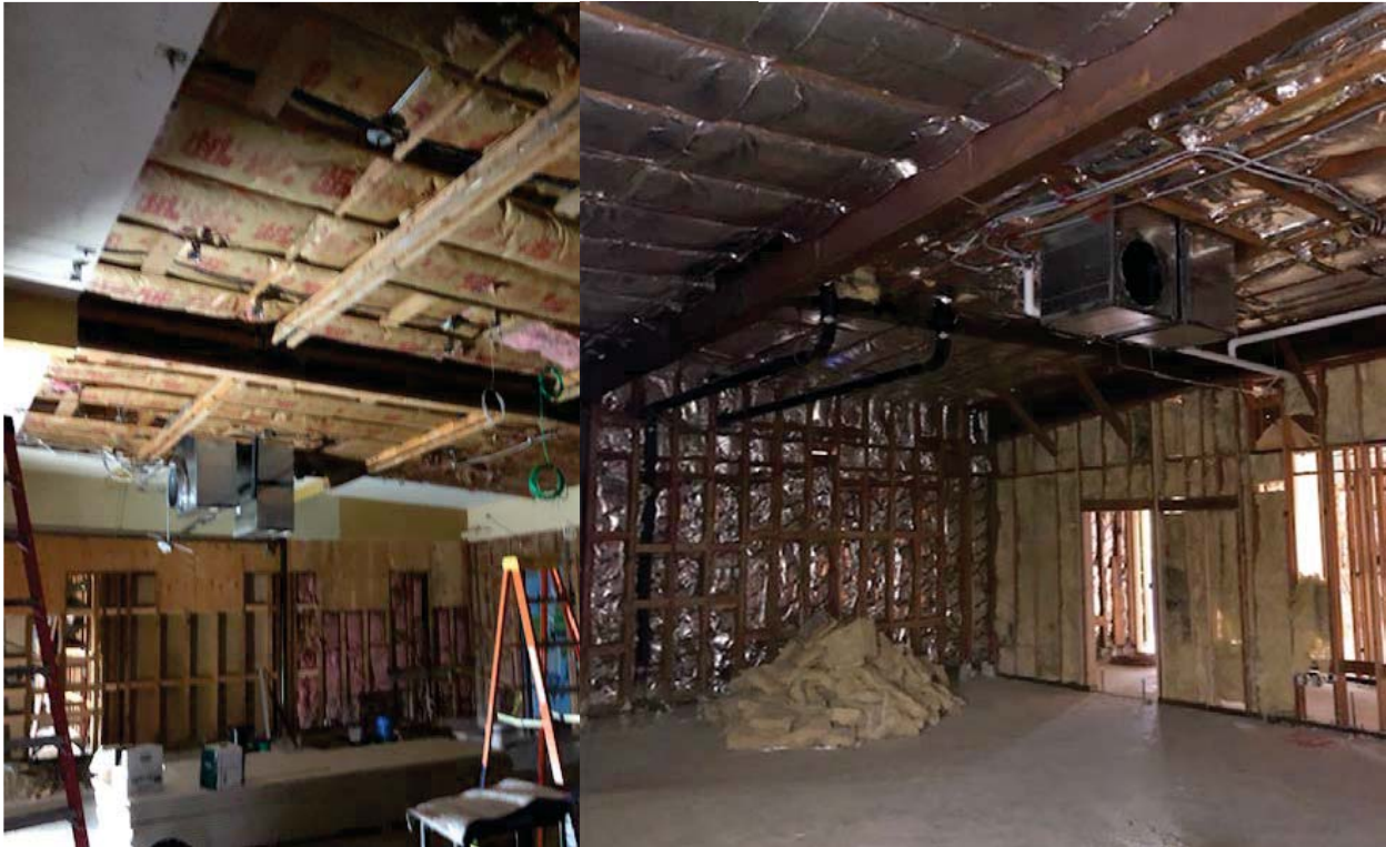
A Building Class Rooms 103, 104 and 105
