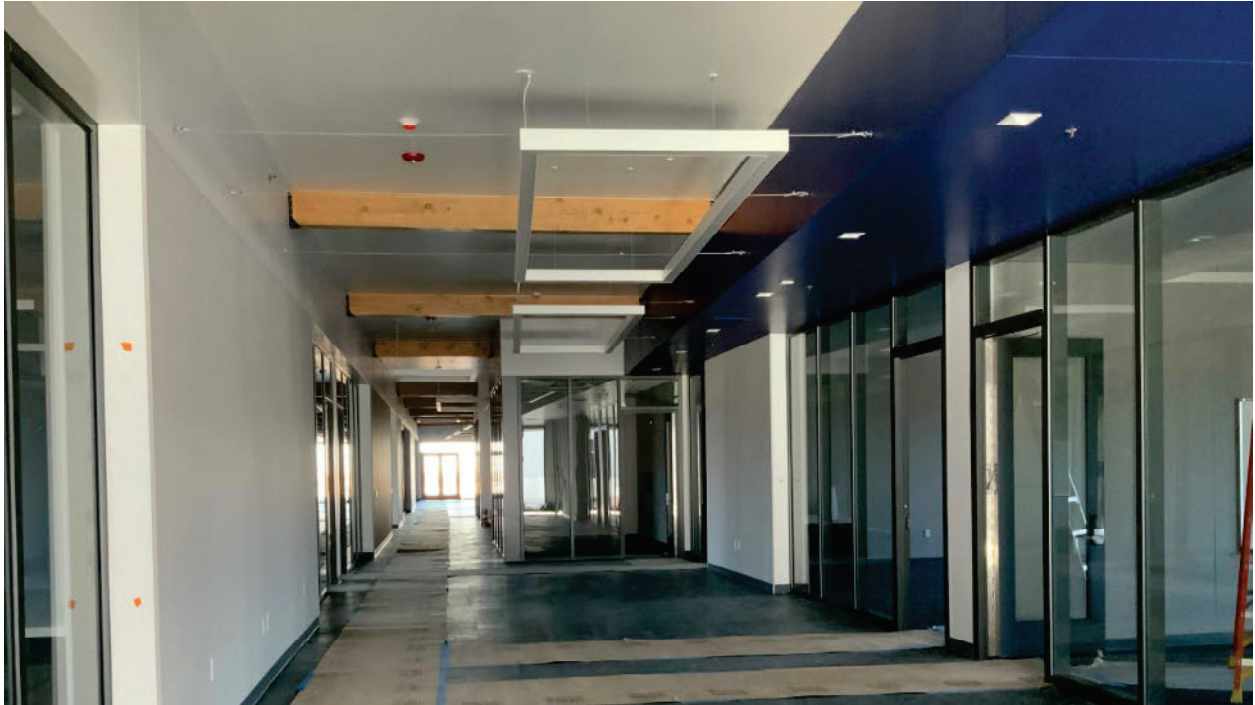
Interior Hallway/Collaboration Space
