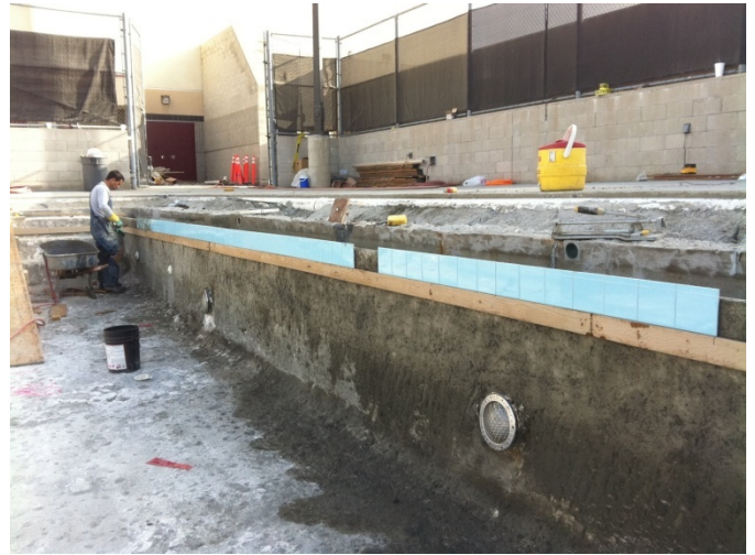
2. Waterline tile installations.
