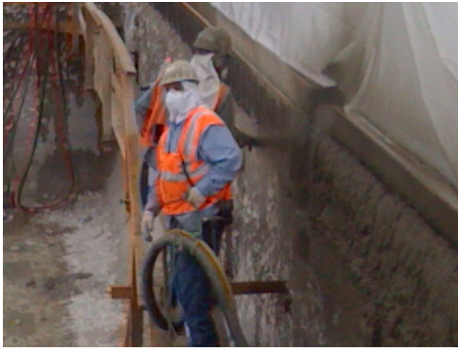
1. Shotcrete at new gutter lip.
