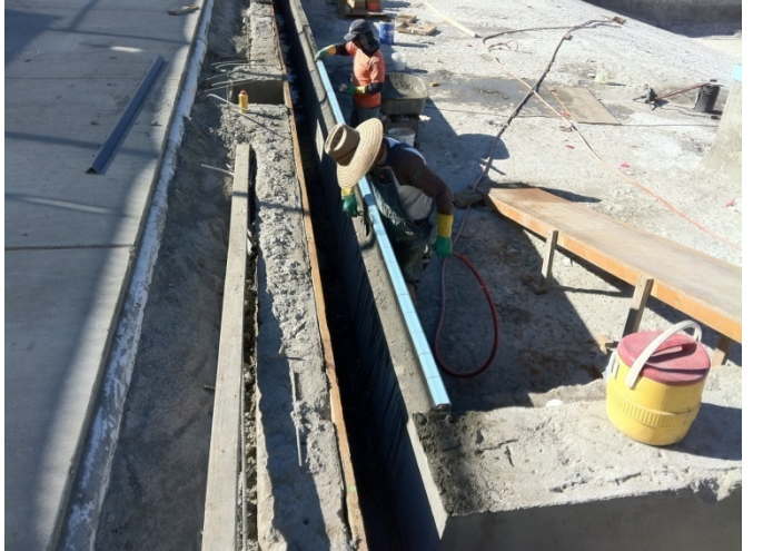
4. Gutter lip cap tile installations.
