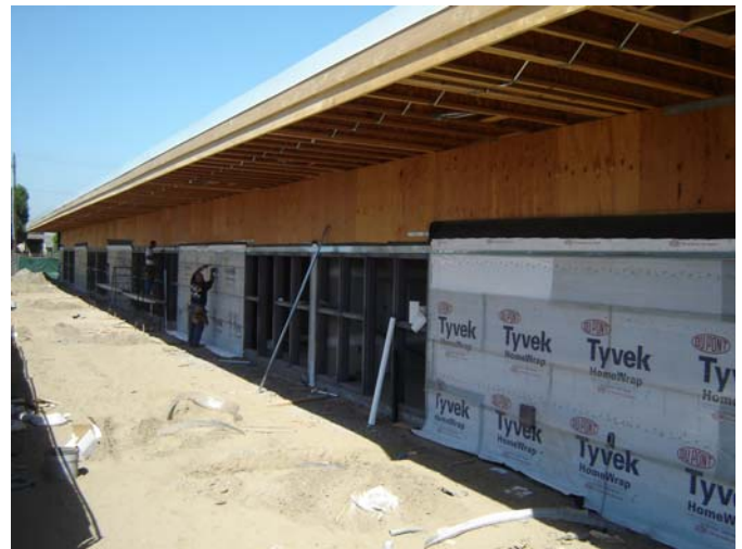
2. Installation of exterior wall moisture barrier.
