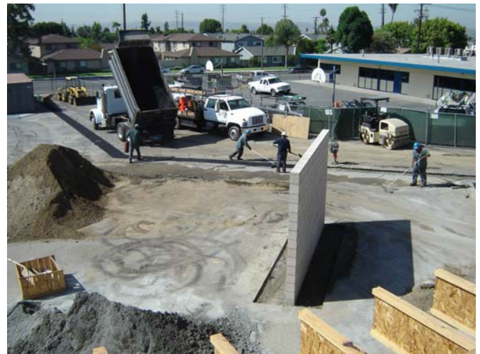
2. Completed concrete stemwall footings.
