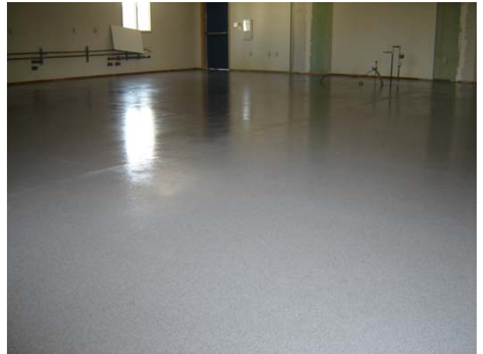
2. New epoxy flooring in Relocatable Classroom.
