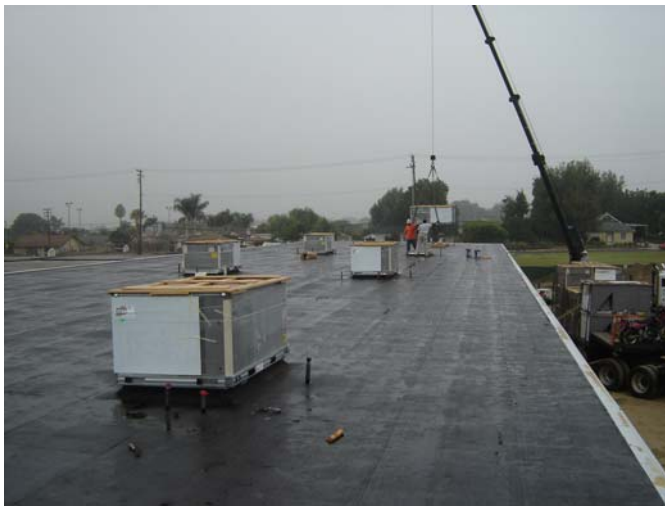
1. Installation of rooftop a/c units.
