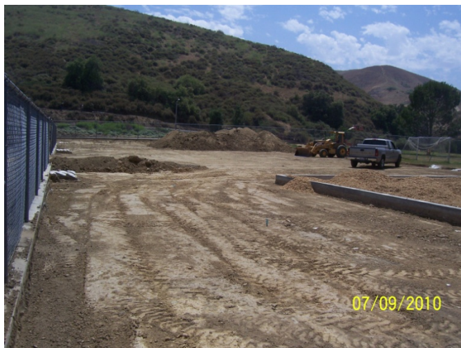
3. Butterfield Ranch – Grubbing and Grading Complete.
