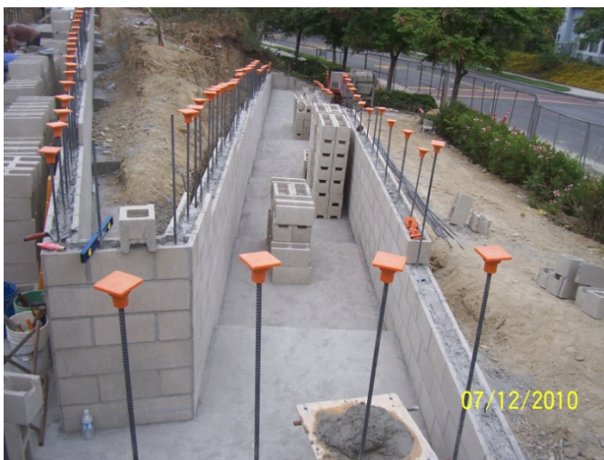
3. CMU Wall In Progress. First Grout Lift Complete.
