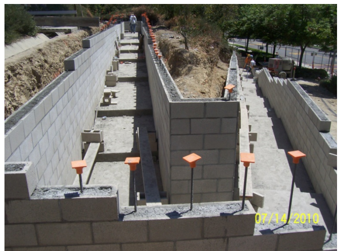
4. CMU Wall Complete and Fully Grouted..
