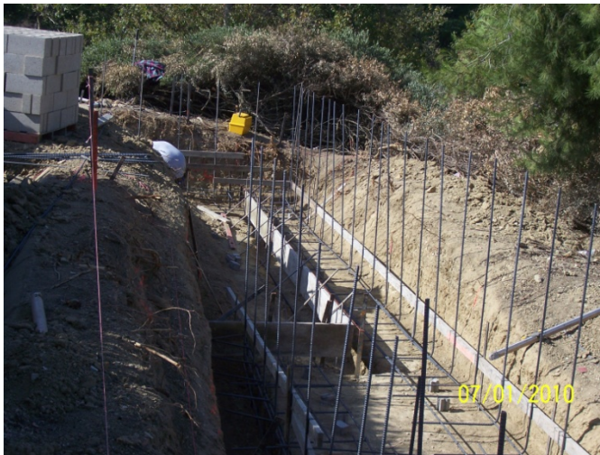
1. Footings Formed and Rebar Installed.
