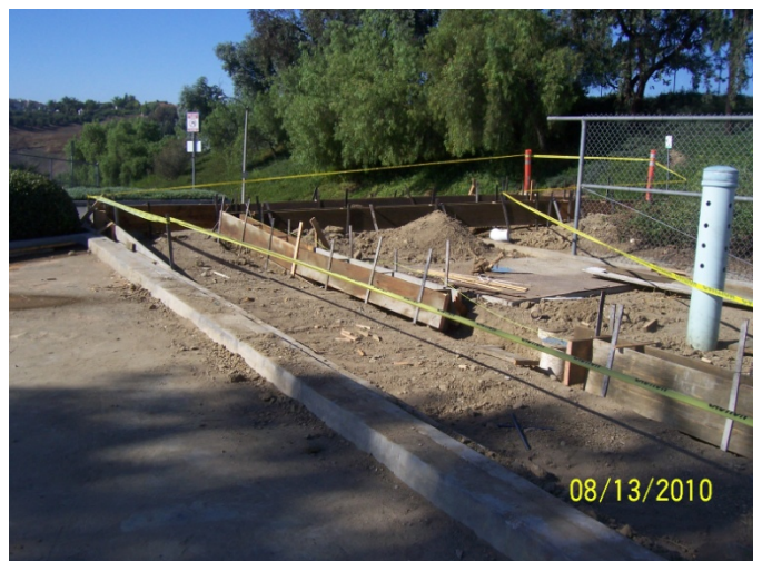
4. Rolling Ridge – Ramp ready for concrete pour.
