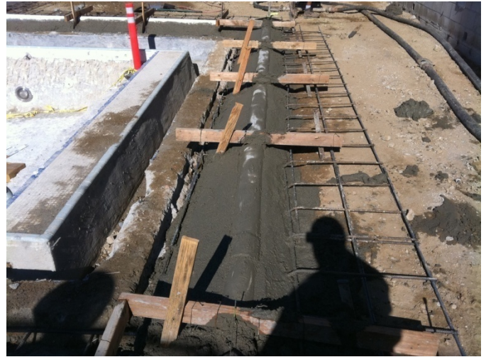
2. Slot drain installation.
