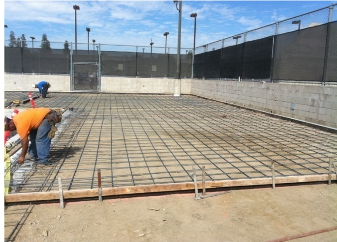
4. Rebar installations @ concrete deck.
