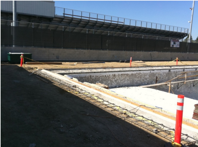
3. Grading for concrete deck pour.
