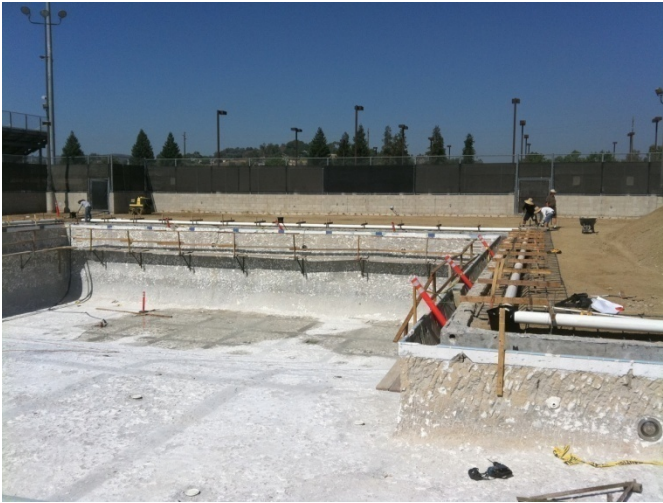
1. Existing plaster and concrete deck have been demolished.
