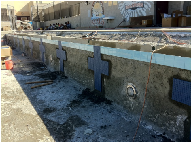
3. Wall target installations.
