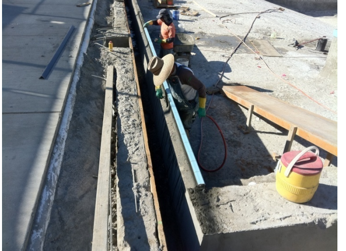
4. Gutter lip cap tile installations.
