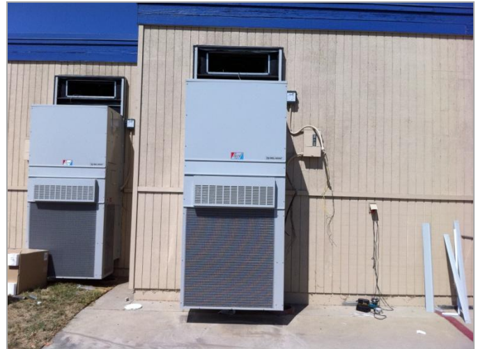
2. Installation of new wall mounted heat pumps and isolation curbs in preparation for equipment guards.
