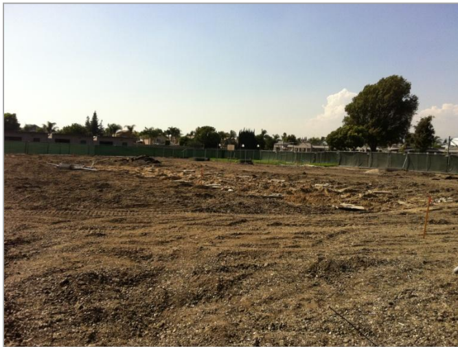
1. Site preparation for over excavation.
