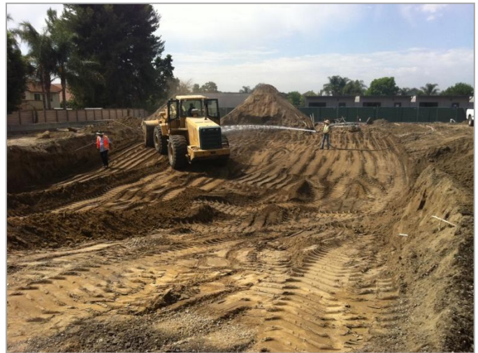
2. Over excavation at the south end of the site.
