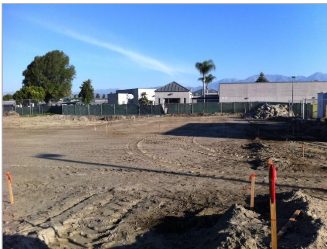
3. Certified and compacted building pad.
