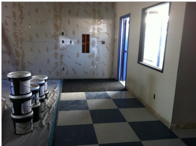
3. Newly installed flooring composed of vinyl composite tile and entry mat geo carpet.
