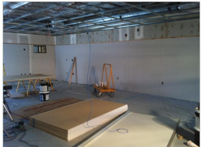
4. Lower vinyl pinboard installation in preparation for eno smart boards, map rail, upper vinyl pinboard and markerboard placement.
