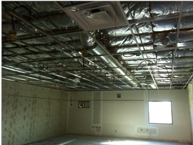
1. Placement of new ceiling tile grid system, roof insulation, and diffusers in preparation for acoustical ceiling tile.
