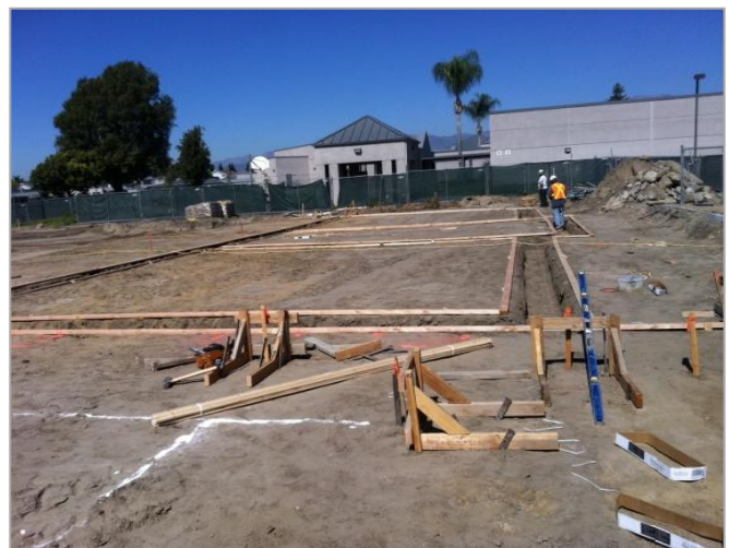
4. Trenching for underground utilities, and formwork for building footings.
