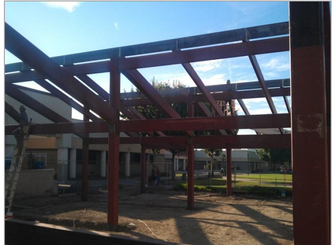
2. Placement of structural steel in preparation for welding.
