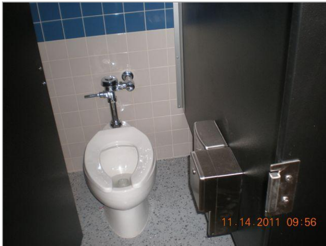
1. Completed toilet partition, toilet, and toilet paper dispenser installation.
