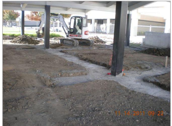
2. Completed grade beam installation.
