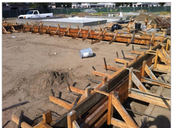
4. South footing formwork.
