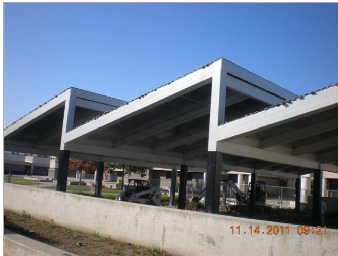
1. Installation of metal roofing.
