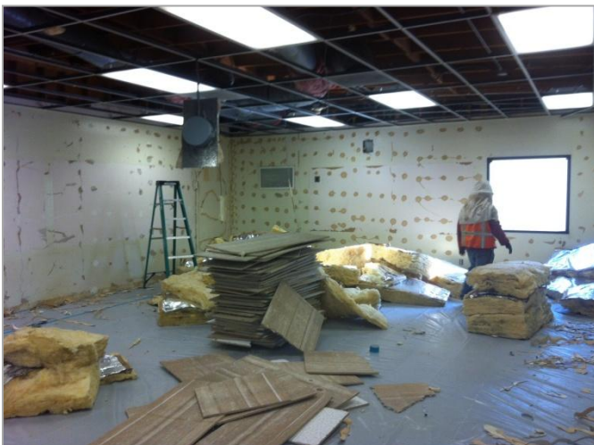
3. Selective demolition of existing ceiling tile, pinboard, light fixtures, insulation, and blinds.-Phase Three
