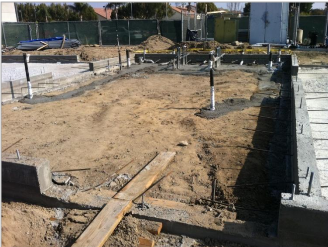
3. Underground plumbing complete.
