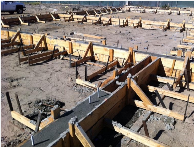
1. Footings and stem walls poured at east and west buildings.
