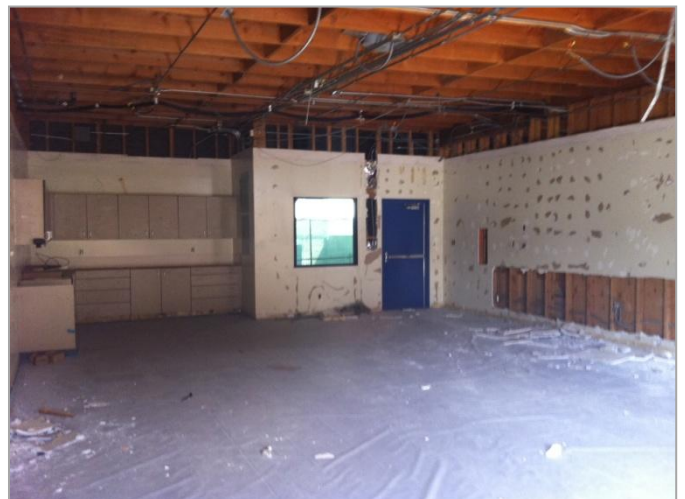
4. Electrical rough in for preparation of new electrical receptacles, interactive whiteboard, light fixtures, and pinboard.-Phase Three
