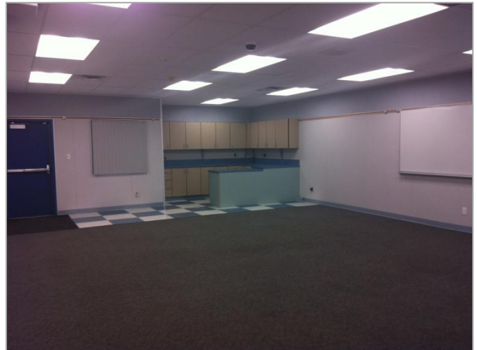
2. Completed new ADA accessible casework, countertops, back splashes, vinyl composite tile, and entry carpet.-Phase Two
