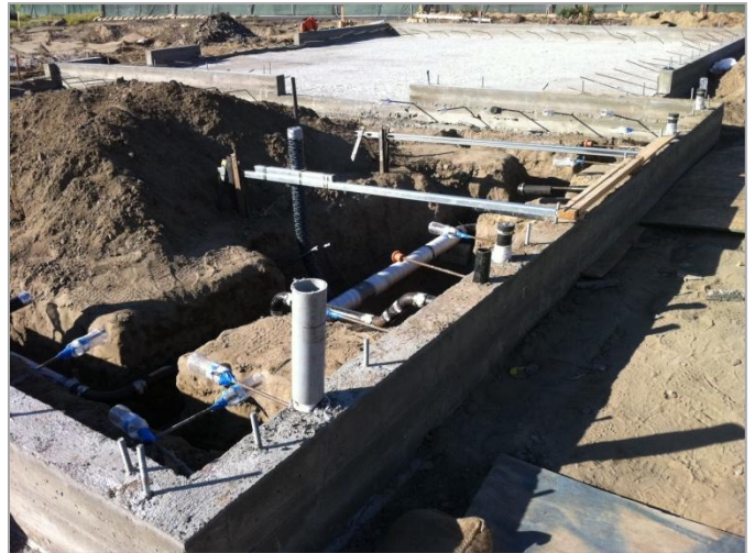
2. Crushed base and underground MEP in progress.
