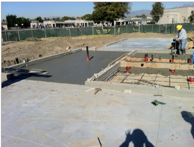
3. Final West Building slab on grade pour.
