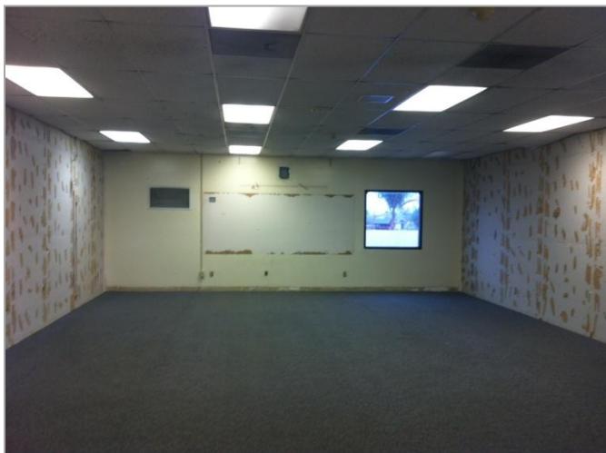
3. Selective demolition of existing pinboard, blinds, and base. -Phase Four
