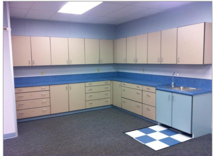
2. Completed new ADA accessible casework, countertops, back splashes, vinyl composite tile, and sink.-Phase Three
