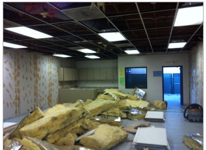
4. Selective demolition of ceiling tile grid, ceiling tile, light fixtures, insulation, and casework.-Phase Four
