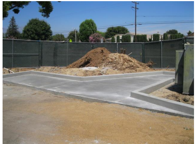
2. Completed concrete placement for accessible curb and ramp.
