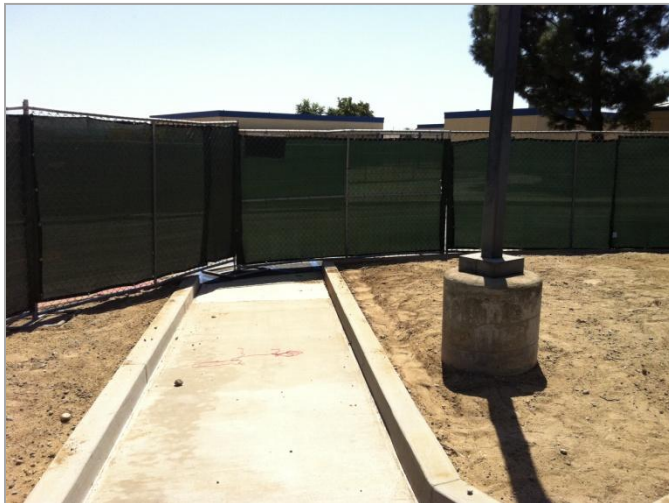
1. Completed accessible concrete pathway, concrete curbs, and truncated domes.
