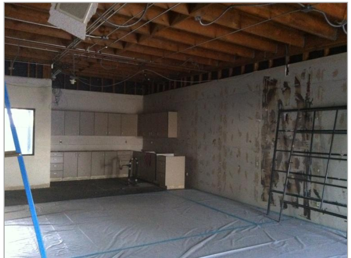
4. Demolition of existing ceiling tile and lights in preparation for new wall coverings, light fixtures, and ceiling tile and grid.
