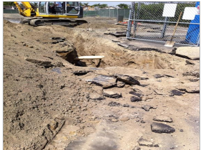
4. Existing fire line to be upsized.
