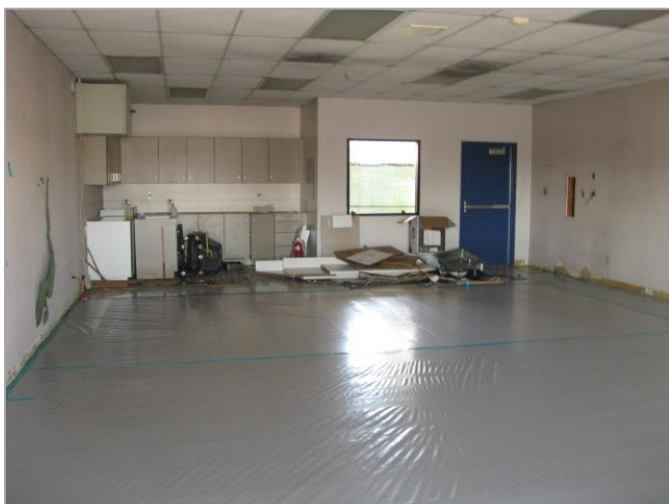
3. Demolition of existing countertops, sink, and protection of existing carpet.
