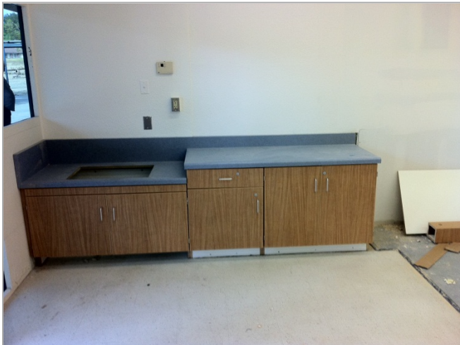
1. Casework installation in progress.
