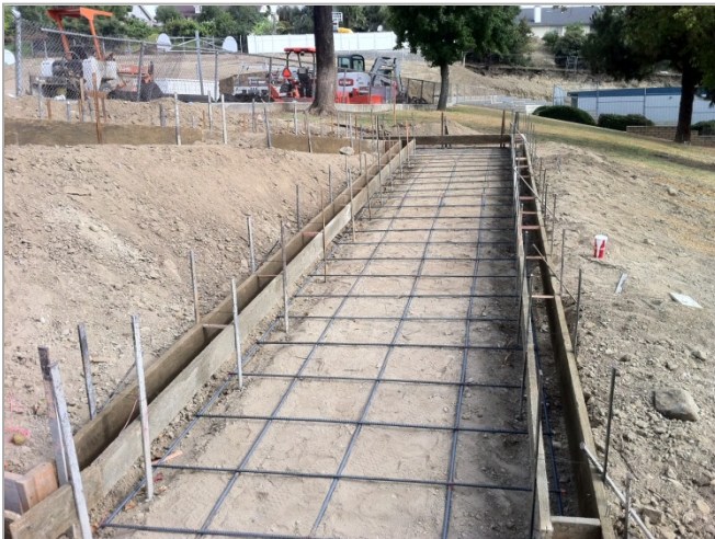
1. Switchback ramp forming and rebar in progress.
