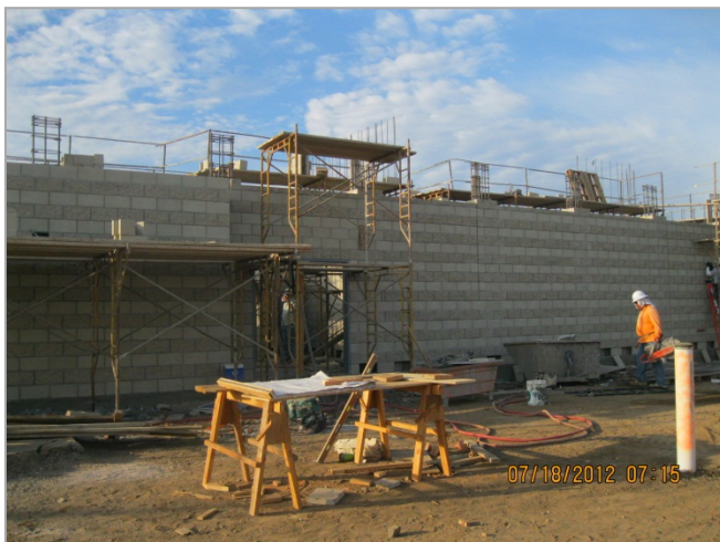
3. Mechanical Building Masonry first lift ready for grouting
