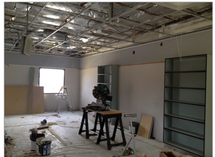
4. Completed pinboard, insulation, ductwork, and casework in preparation for eno board, ceiling tile, base, and blinds.-Phase Nine
