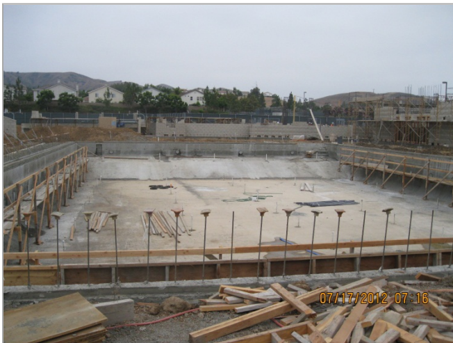
1. Pool Floor, Walls, Stairs and Gutter Shotcrete/Concrete done.
