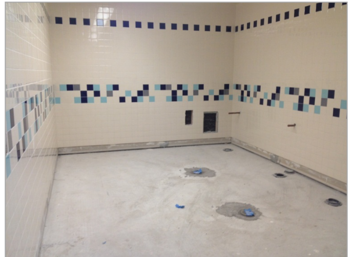
2. Completed ceramic tile and grout placement at student restrooms in preparation for epoxy floor placement.-Phase Nine
