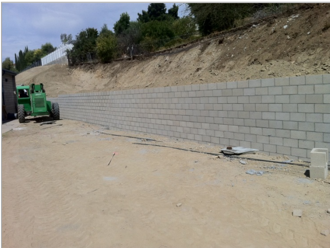
3. CMU retaining wall in progress.
