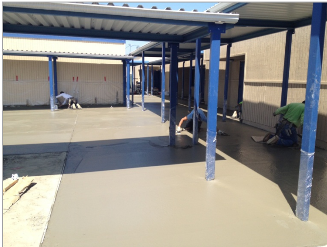
1. Completed concrete placement and finish work at Building C and O for ADA grade requirements.-Phase Nine
