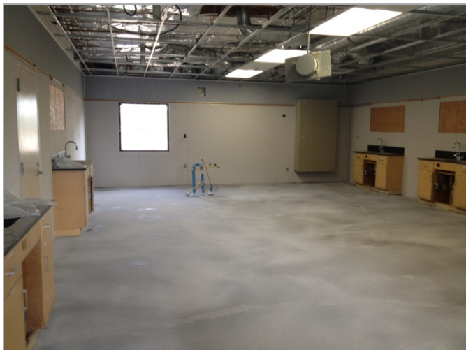
3. Installation of pinboard, ceiling tile grid, and ductwork, in preparation for epoxy floors and ceiling tile placement.-Phase Nine
