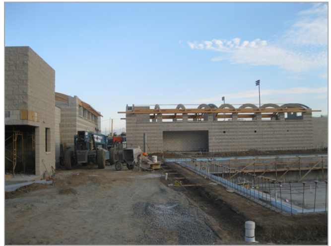
2. Building Masonry and Glue-Laminated Beams Complete
