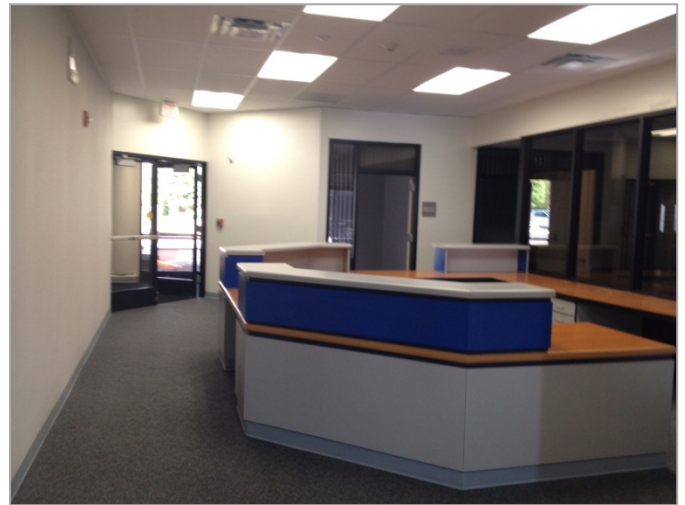
2. Placement of new reception desk, pinboard, light fixtures, ceiling tile grid, carpet, and ceiling tile.-Office
