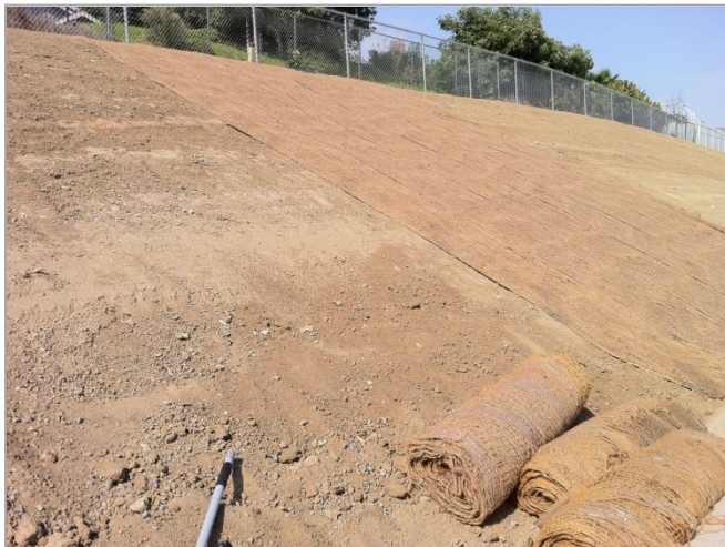
3. Jute installation on slope.
