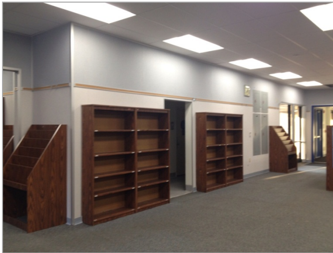
1. Completed casework, ceiling tile grid, light fixtures, ceiling tile, base, and pinboard.-Library
