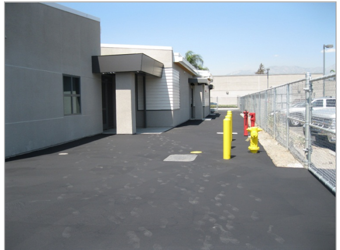
2. Asphalt Paving and Slurry Seal Complete.
