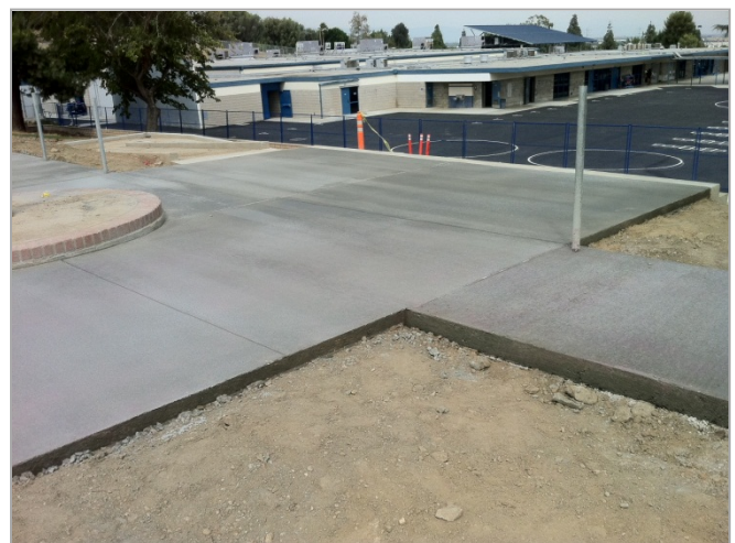
4. Concrete at field area walkway placed.
