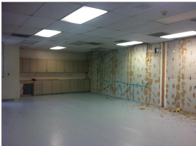
3. Installation of floor protection and selective demolition of existing pinboard, countertops, and base.-Phase Five
