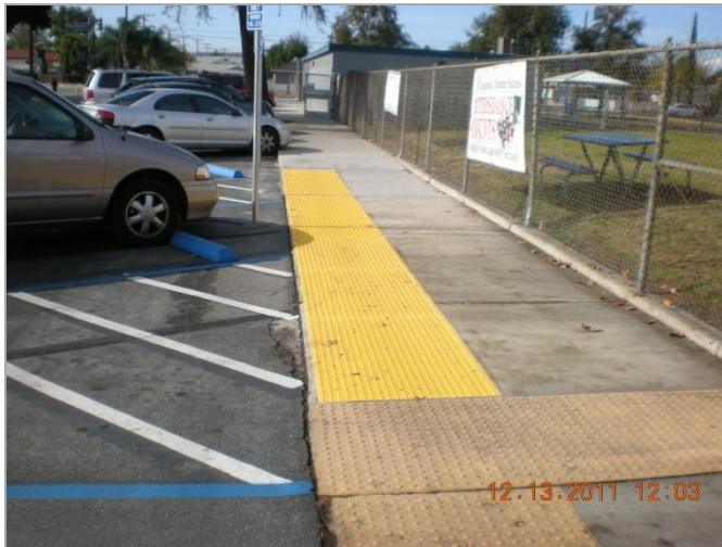
1. Completed truncated dome installation for new ADA requirements.
