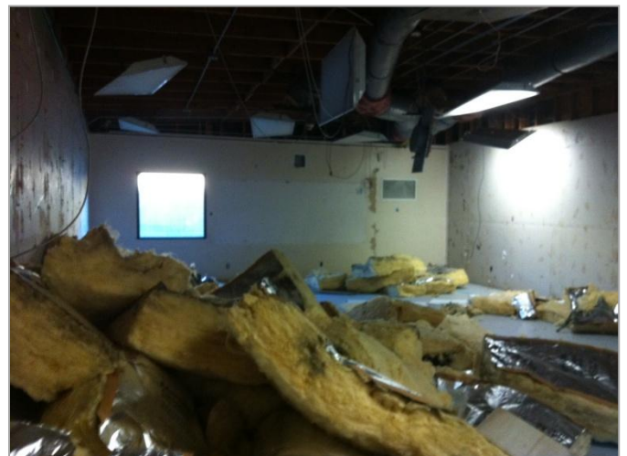
4. Selective demolition of ceiling tile grid, ceiling tile, light fixtures, insulation, and pinboard.-Phase Five
