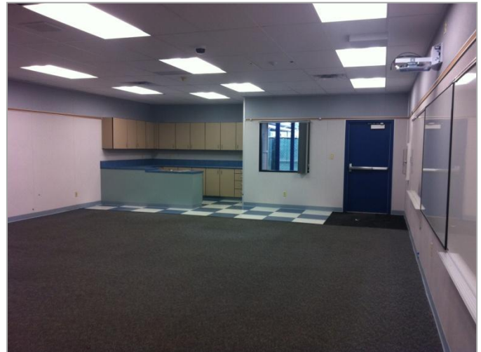
2. Completed new ADA accessible casework, countertops, back splashes, vinyl composite tile, and sink.-Phase Four
