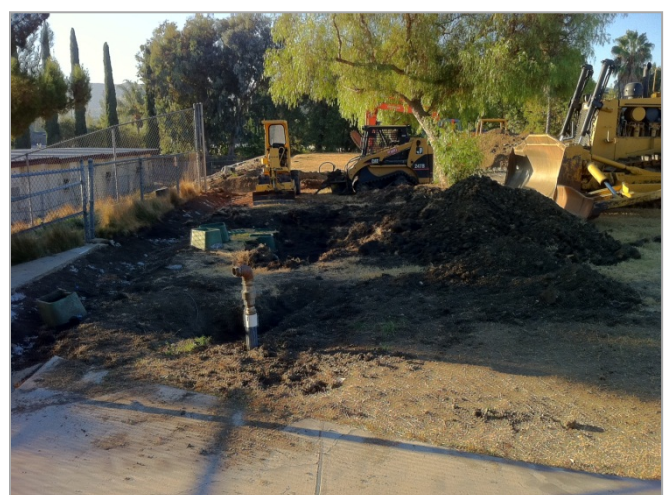
4. Underground utilities and swale removal and rework in progress.
