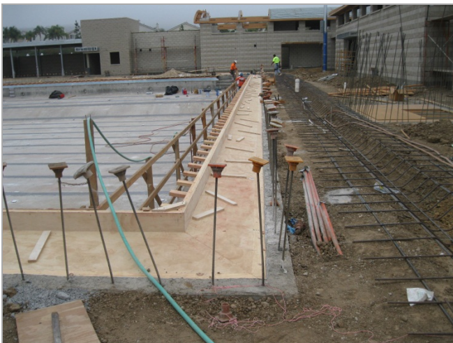
1. Pool Tile Installation Complete w/ Deck Forming In Progress
