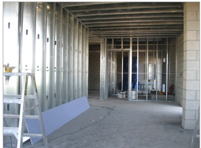
2. Building Metal Stud Framing In-Progress
