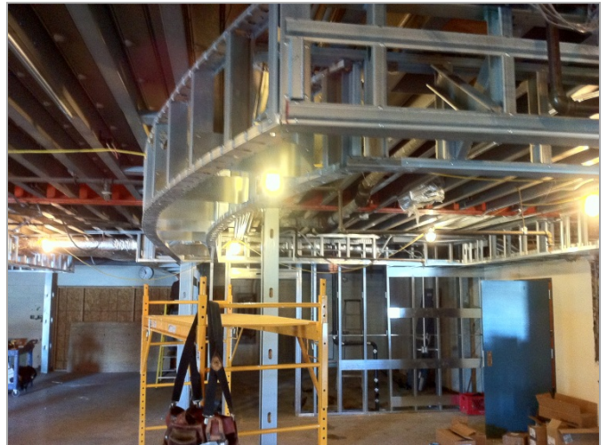
2. Metal-stud soffit framing and MEP rough-in at new Library.
