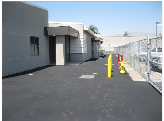
2. Asphalt Paving and Slurry Seal Complete.
