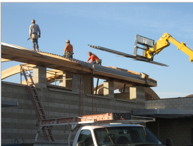
3. Building Metal Decking Installation In-Progress
