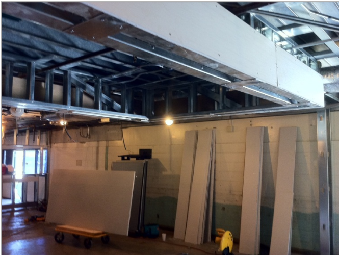
1. Drywall at dropped soffits in progress at Library.
