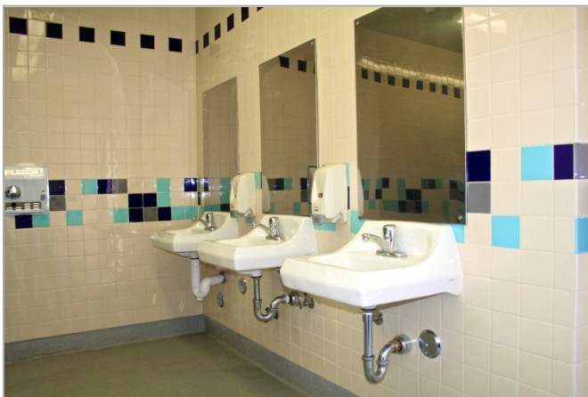
3. Placement of new ceramic tile, lavatories, mirrors, hand dryer, soap dispensers and epoxy flooring.
