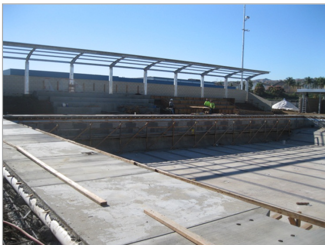
3. First bleacher section is poured
