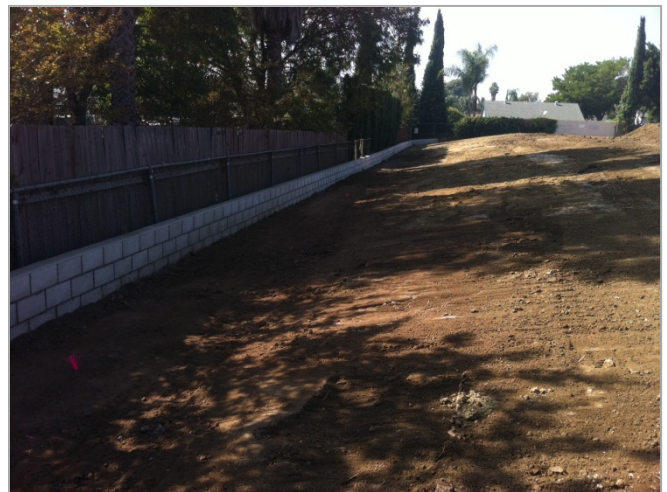
2. South slope and CMU splash wall complete
