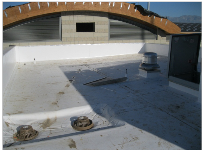
2. PVC roofing is complete and the building is dried-in
