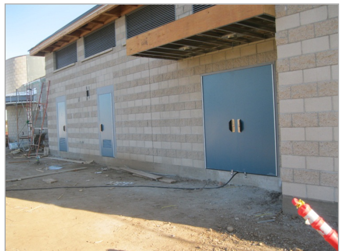
4. Louvers and exterior doors are installed
