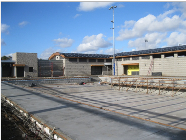
1. Pool inner deck is poured
