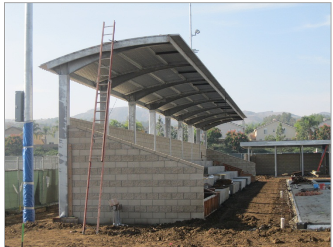
2. Bleacher canopy decking is installed
