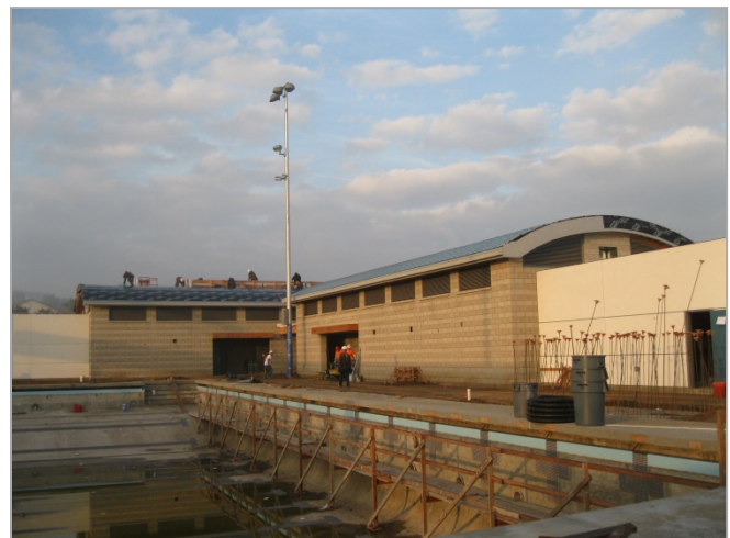
4. Building plastering complete & standing seam roofing in progress
