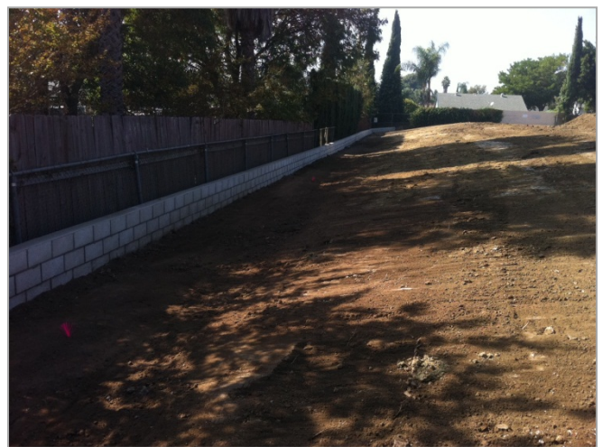
2. South slope and CMU splash wall complete
