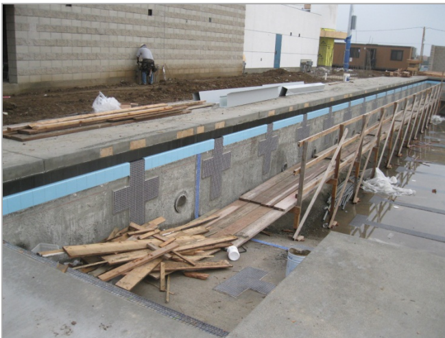
1. Pool gutter and inner deck are poured and formwork is stripped
