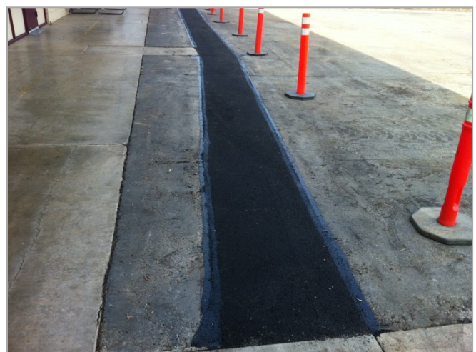
4. Main irrigation line tied in and patched back.
