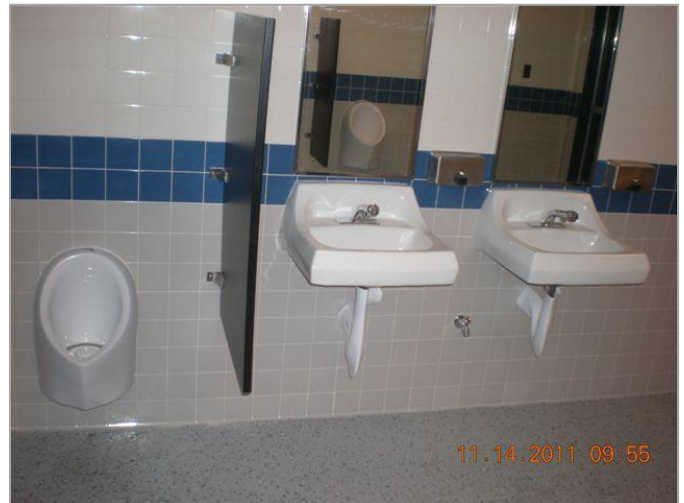
2. Installation of new sinks, mirrors, waterless urinals, and partitions.
