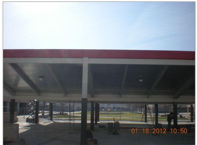
2. Completed grade beam installation and standing seam metal roof placement.
