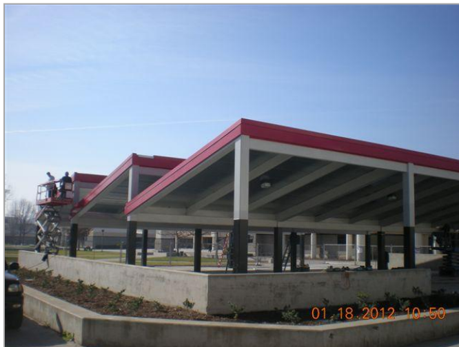
1. Placement of concrete curbs, planters, and landscaping shrubs and mulch.
