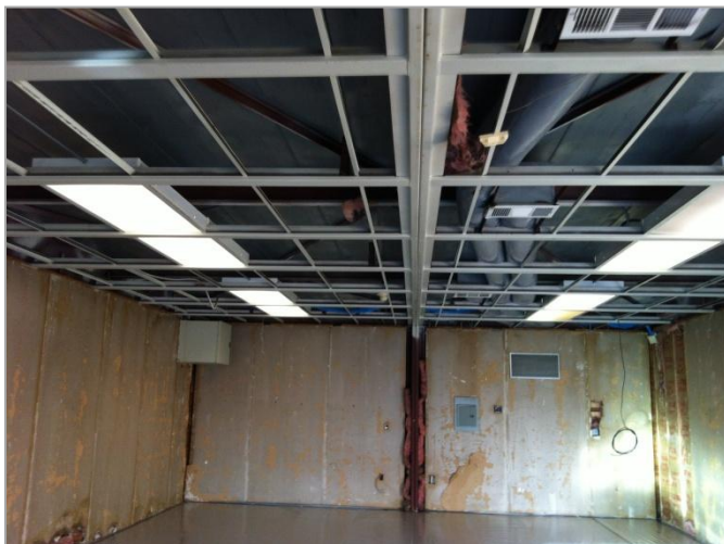
3. Installation of floor protection and selective demolition of existing pinboard, base, ceiling tile and light fixtures.-Phase Six
