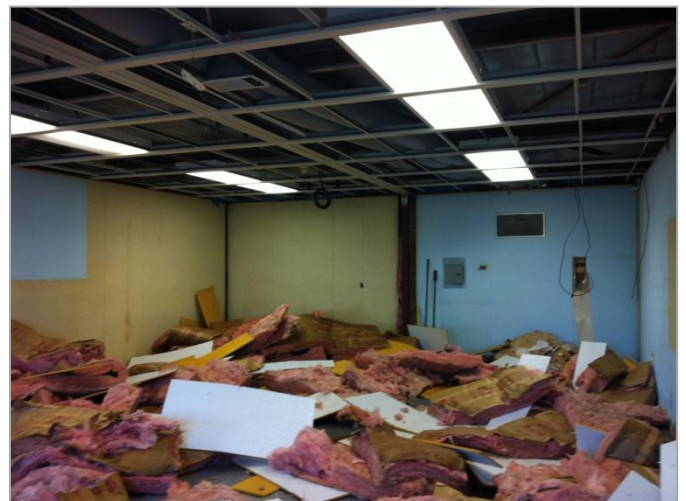
4. Selective demolition of ceiling tile, insulation, light fixtures, and pinboard.-Phase Six
