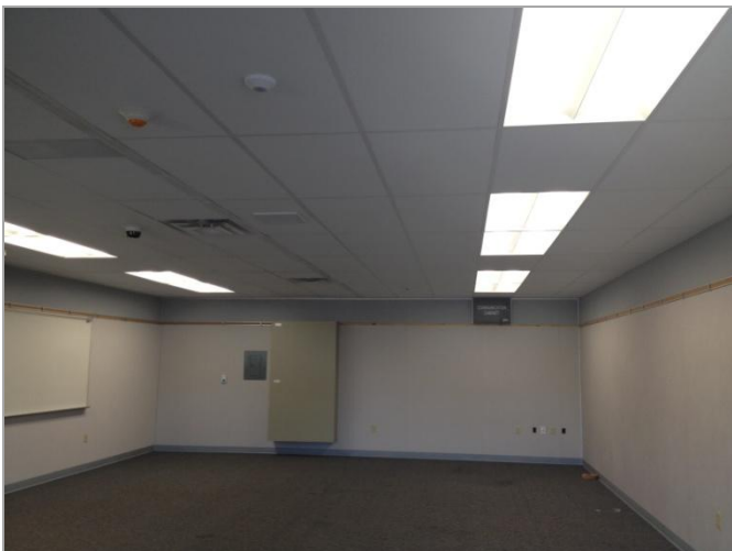
3. New light fixtures, ceiling tile, return air plenum, pinboard, base, and maprail at the Band Room.-Phase Six
