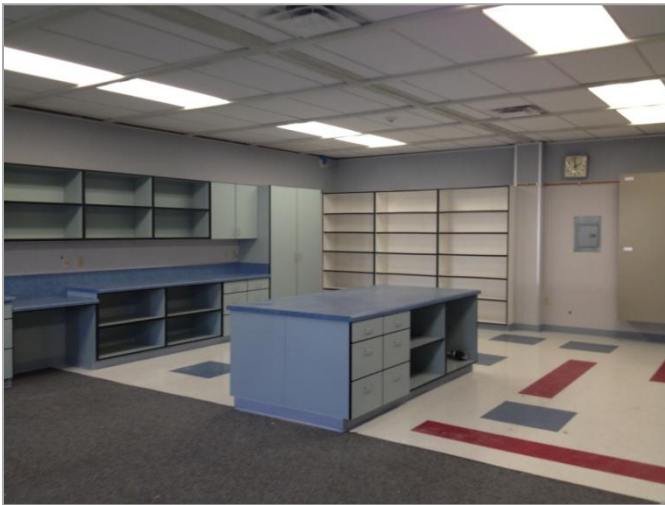
1. Completed new casework, countertops, backsplash, pinboard, and vinyl composite tile flooring at the Teachers' Workroom.-Phase Six
