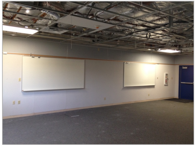
2. Installation of new pinboard and markerboards, in preparation for the new interactive whiteboard.-Phase Eight
