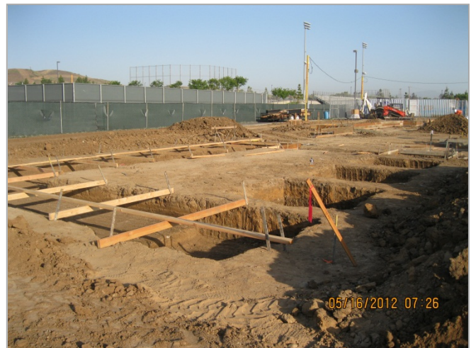
4. Building Mat Slab and Footings being prepared.
