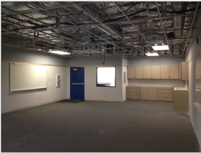
1. Completed pinboard, ductwork, ceiling tile grid, and markerboard installation.-Phase Eight
