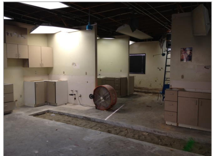
4. Selective demolition of existing ceiling tile, insulation, light fixtures, flooring, and countertops.-Phase Nine
