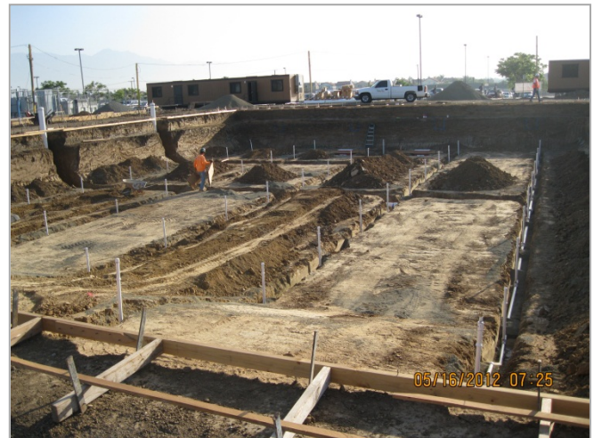
2. Pool Underground Piping Roughed-In and Under Test.
