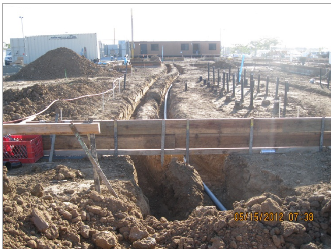
3. Building Underground Electrical and Plumbing in progress.
