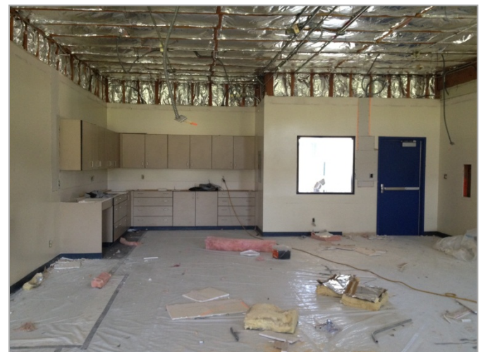
4. Completed electrical rough in, drywall patch, and insulation for placement of new ductwork, pinboard, and ceiling tile.-Phase Nine
