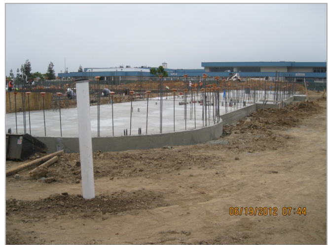
2. Concession Building Mat Slab and Foundations Poured
