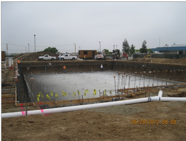
1. Pool Floor Complete and Wall/Gutter Rebar 90% Complete
