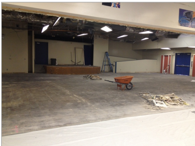
3. Demolition completed of the ceiling tile and grid, sliding glass wall, and vinyl composite tile in preparation for new stud wall.-Phase Nine
