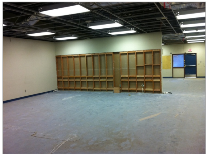
2. Demo complete, blocking in progress.
