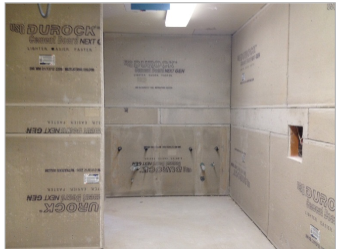
2. Completed electrical and plumbing rough in with placement of cement backer board in preparation for ceramic tile.-Phase Nine
