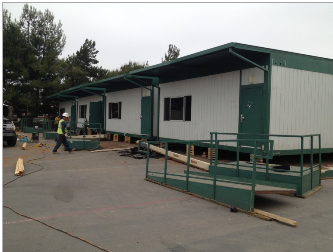
1. Disassembly of the four portable buildings, in preparation for removal and asphalt patch.-Phase Nine
