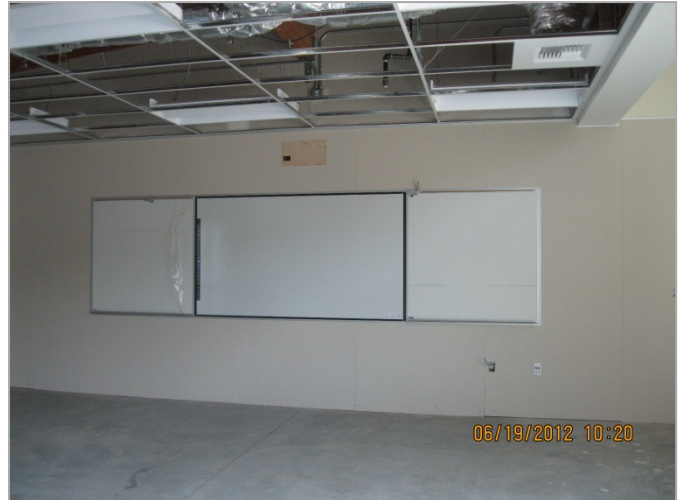
2. Tackboard and Markerboard installation is complete
