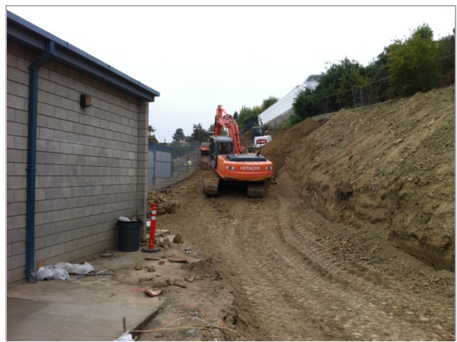
2. Overexcavation and slope grade cuts in progress.
