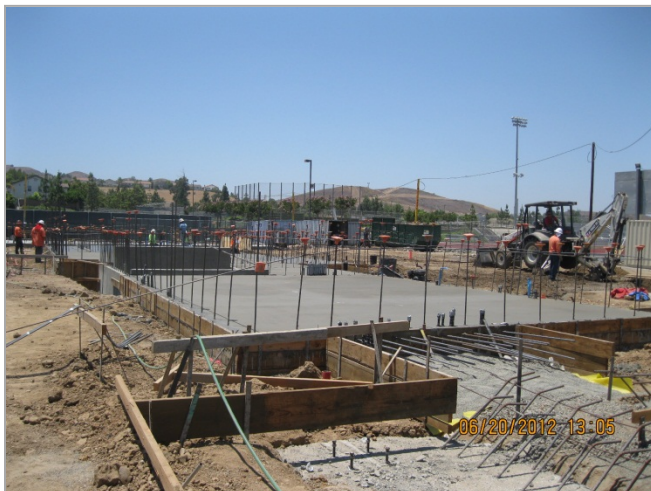
3. Mechanical Building Mat Slab, Pits and Foundations Poured
