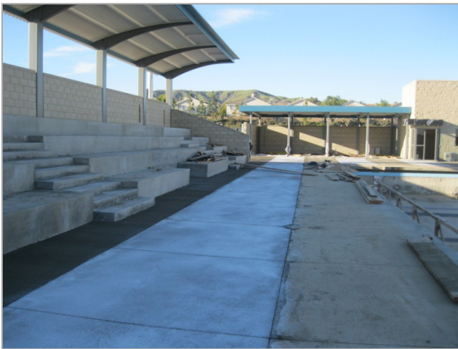
1. Pool decks and bleachers are poured
