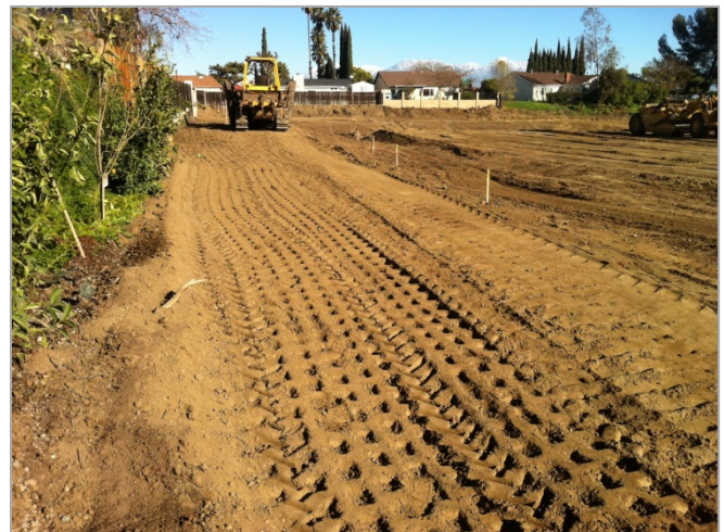
4. Building up slope along northwest property line.
