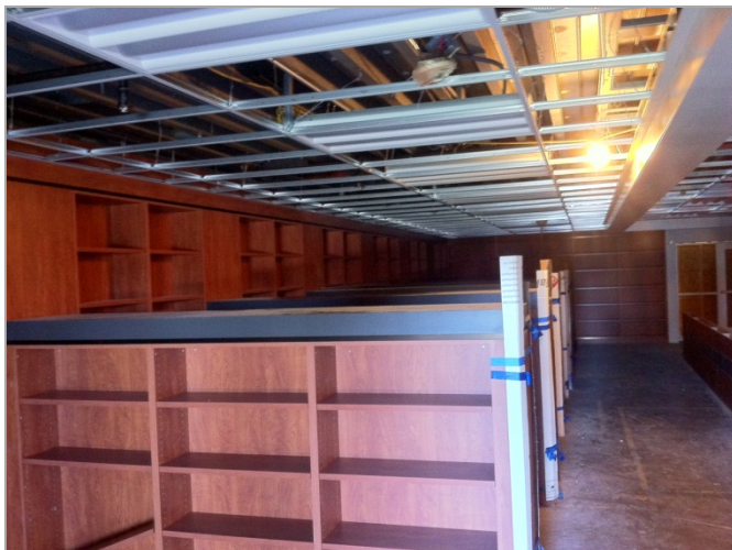
3. Library casework, ceiling grid and light fixture install in progress.
