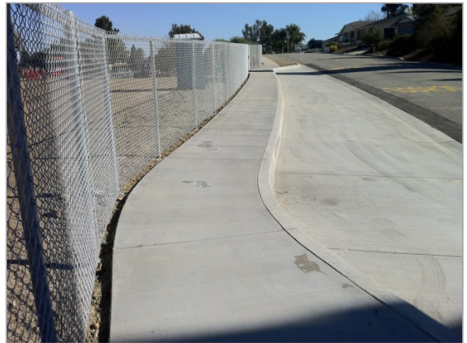
2. Bus drop concrete placed.
