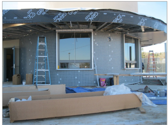
2. Exterior tiling and sheet metal trim/soffit panel installation in progress
