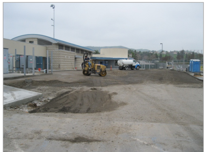
4. Base is installed and asphalt is being placed
