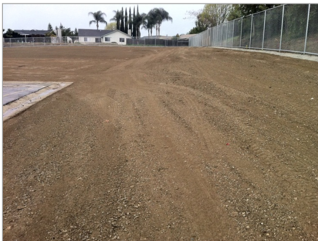
3. North slope complete and ready for hydroseed.
