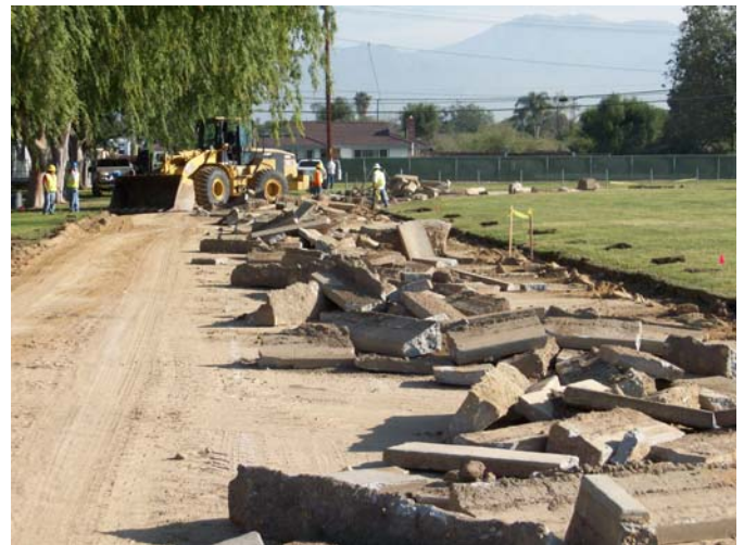
4. Removing existing curb and gutter.
