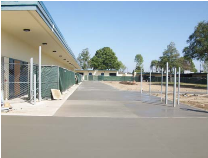
1. New concrete walkway was poured and fence posts were installed.
