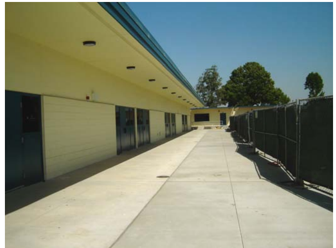
2. Building X: New exterior steel doors and concrete walkway.
