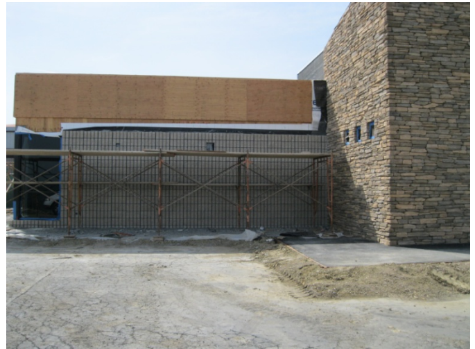
2. Brick veneer and stacked stone installed.
