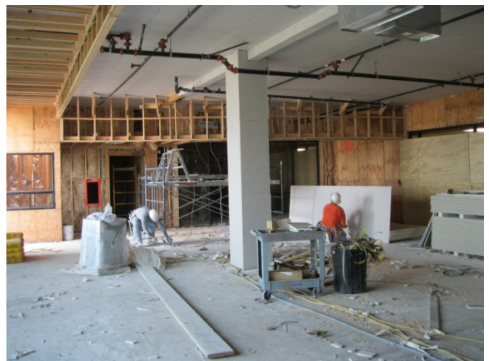
4. Drywall installation in progress.
