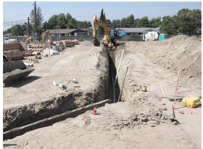
4. Over-excavation for sewer line on-going.
