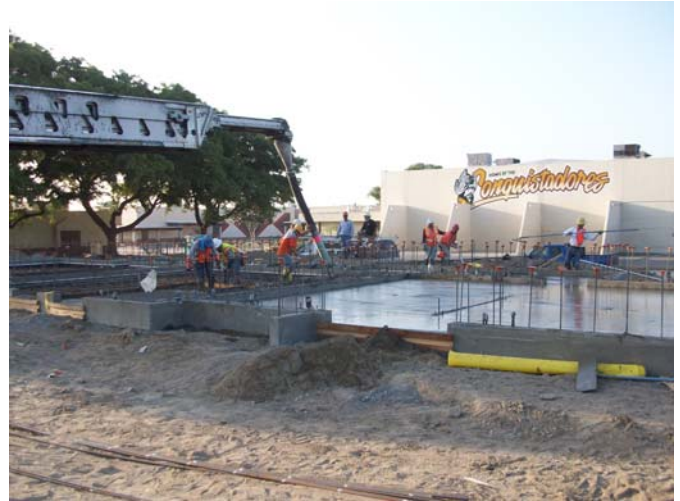
2. Building B- Pouring concrete slab.
