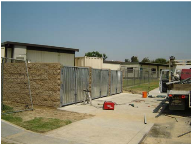
3. New trash can enclosure and trash can washing area on-going.
