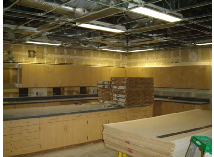
2. Installation of casework and t-bar complete.
