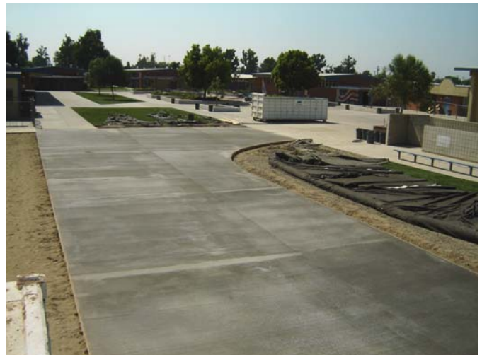
4. New concrete fire lane complete.
