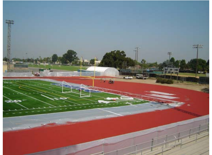
2. Chino HS- Installing tracking lining on-going.
