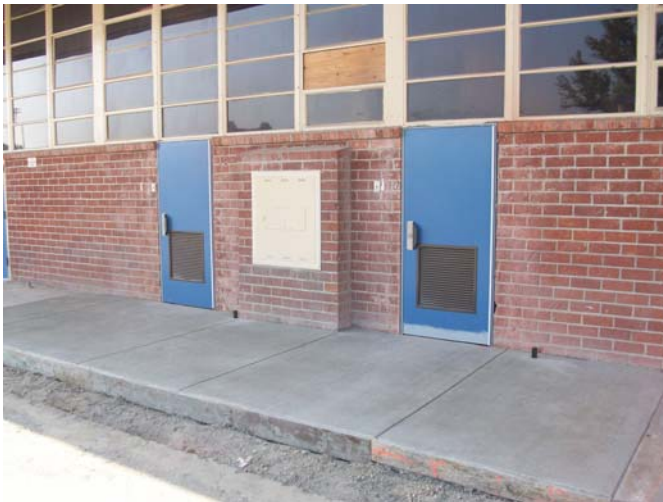
3. Band building- New ADA doors and concrete walkway on-going.
