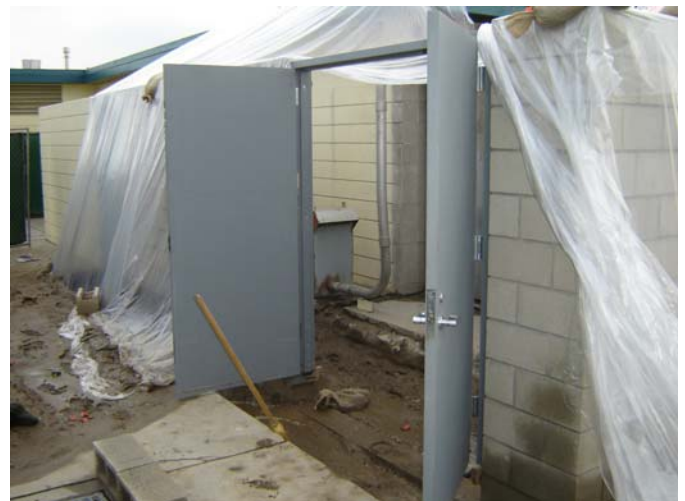
4. New CMU, HM frames & doors were installed at Elect. Enclosure.
