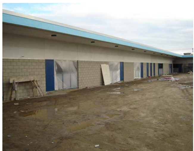
4. West Elev.: Plaster, finish coat was applied & scaffolding removed.
