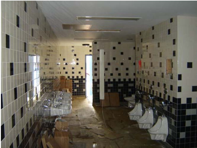
1. Ceramic tile and plumbing finishes at Boy's Restroom.
