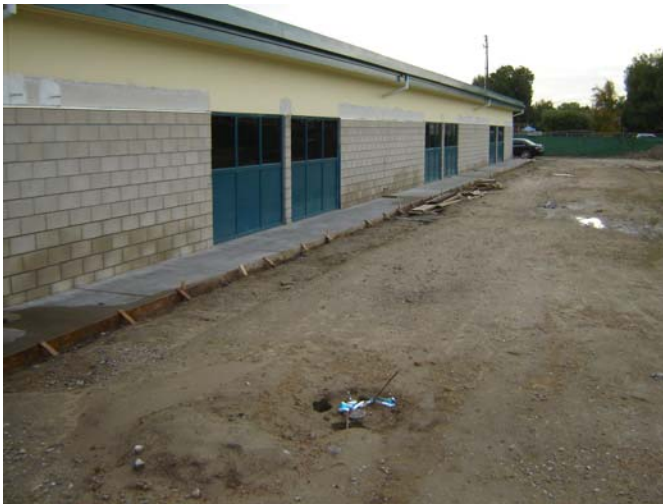
1. Completed concrete walkway at the north side of Bldg. X.
