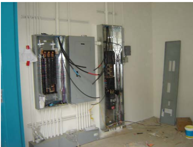
3. Pulling electrical conductors to new MDS room.
