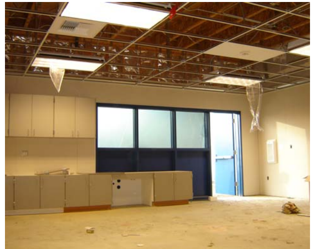
2. New casework, T-bar, lighting and low voltage devices..
