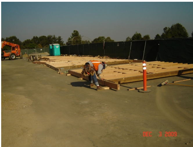
1. Exterior framing in progress.
