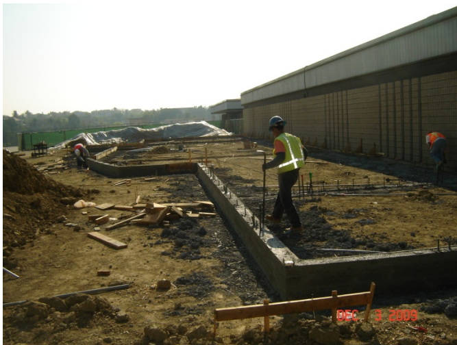
3. Stripping the poured footings.
