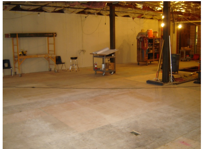
4. Plywood flooring re-installed, drywall hung .
