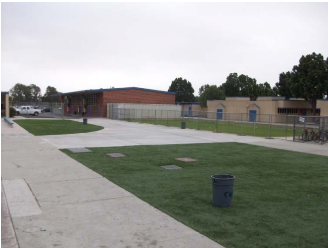
3. New concrete fire lane and hydroseed planter complete.
