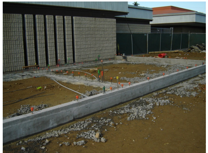
4. Footings stripped, ready for slab-on-grade.
