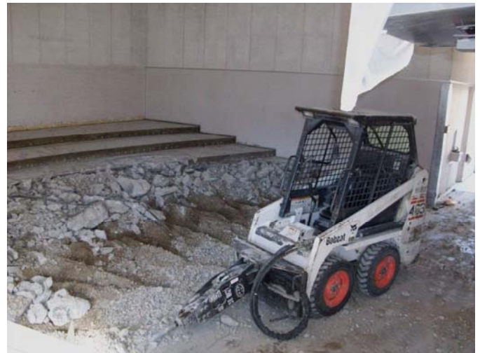
2. Bldg. P- On-going demolishing of existing concrete stairs.
