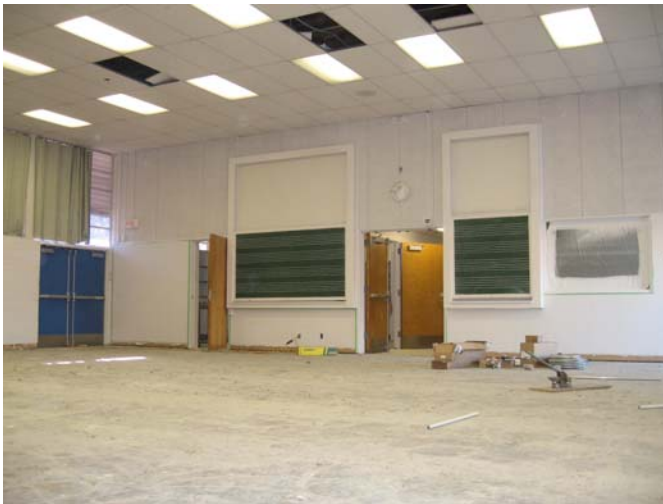
1. Bldg. P- Removed existing carpet, working on painting preparation.
