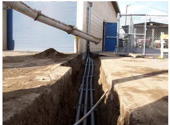
4. Bldg. J- Underground conduits for low voltage systems.
