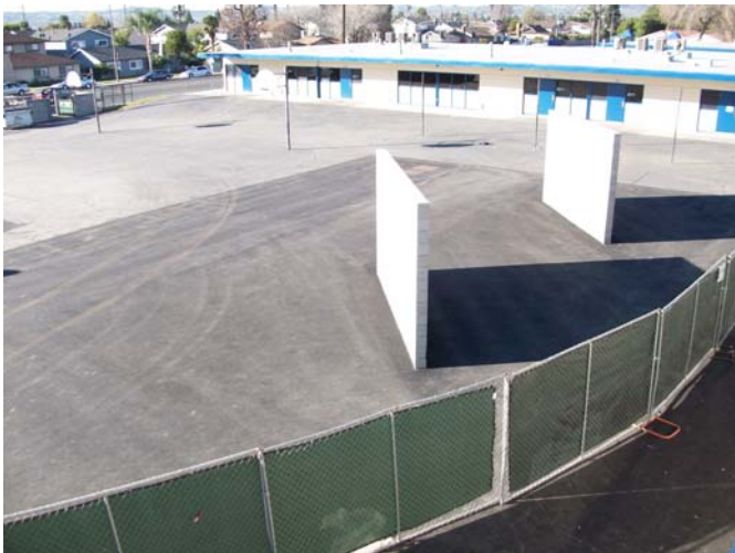
3. New asphalt overlay around the new ball walls.
