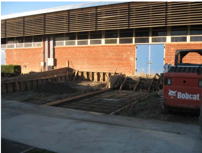
3. Bldg. P- Form work installed for exterior stairs and ADA ramp.
