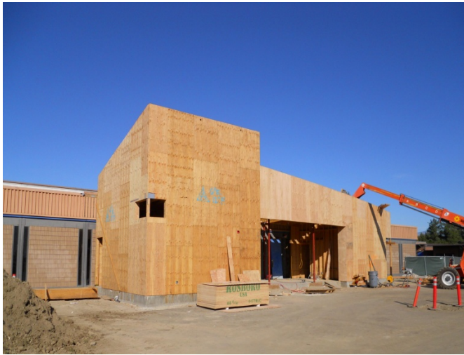
1. Exterior framing complete.
