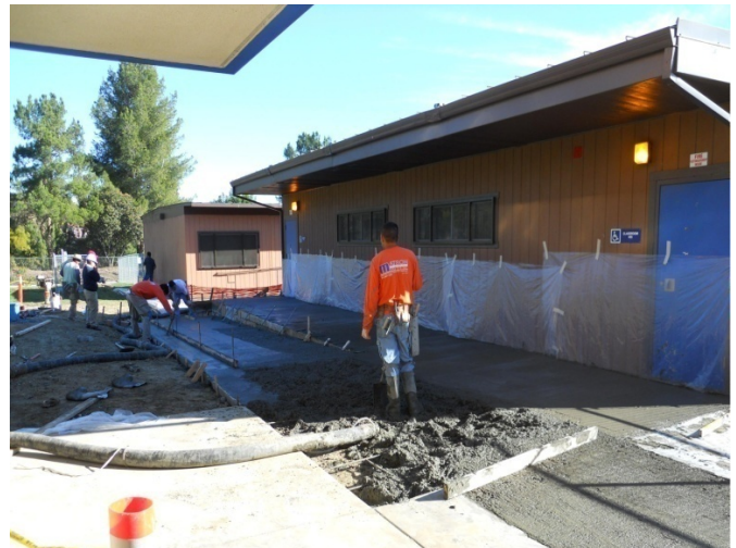
4. Concrete at portables poured during winter break .
