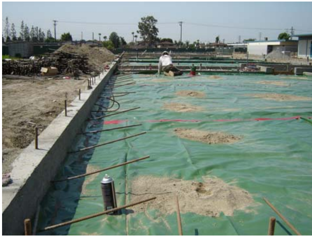
1. Vapor barrier over sand for concrete slab.
