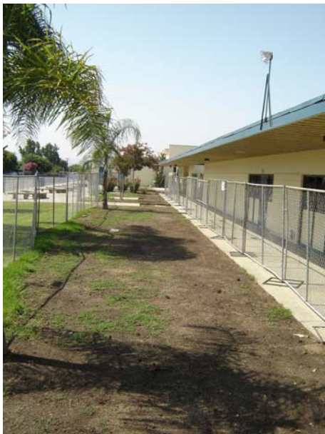
3. Backfilled underground utilities.
