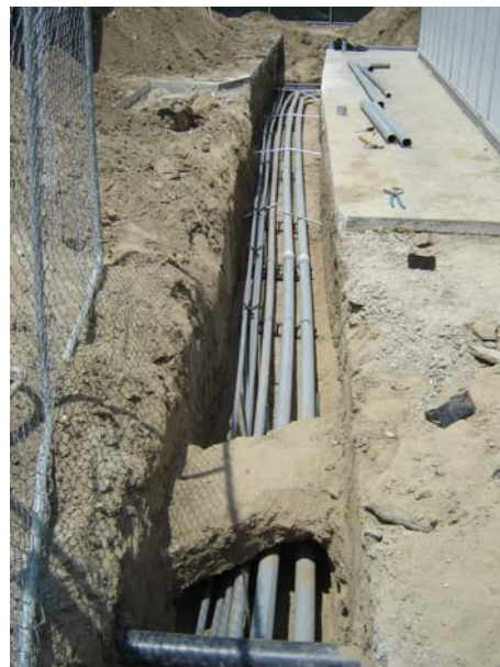
4. Conduits for electrical and low voltage systems.
