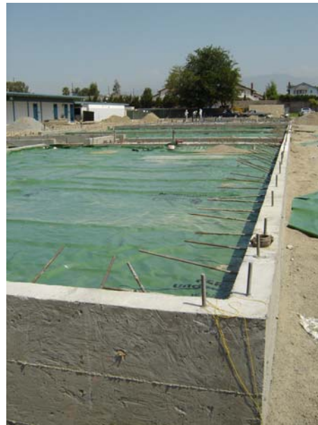
2. Completed concrete stemwall footings.
