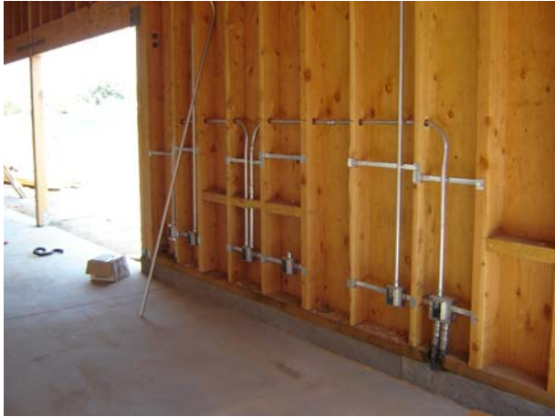
1. Electrical rough-in within classroom walls.
