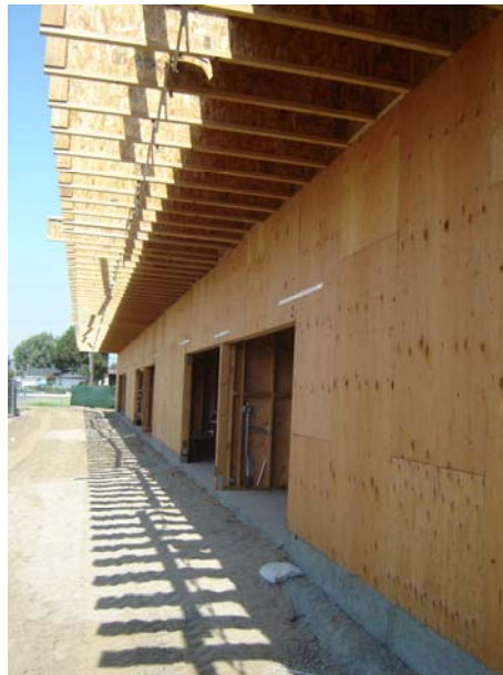
2. Exterior wood framing and sheathing.
