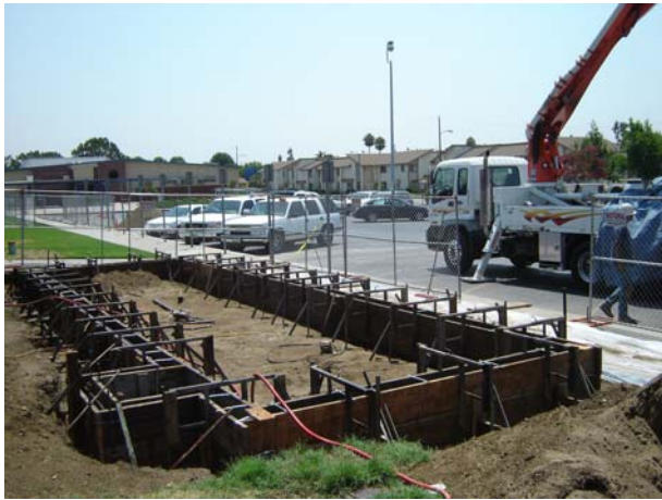
3. Complete formwork and concrete placement at stemwall footings.
