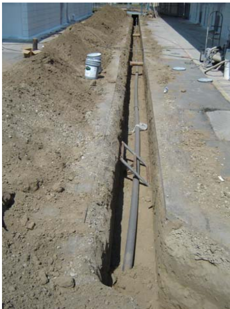
3. Conduit for low voltage systems.
