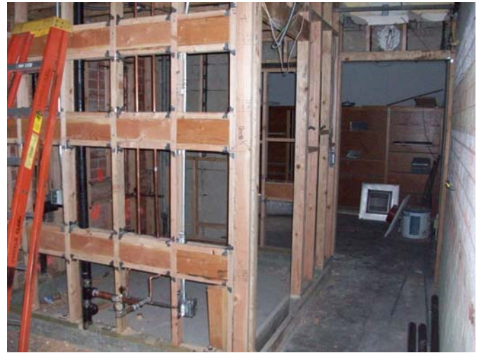
2. Counseling Bldg.- Rough-in electrical and plumbing complete.
