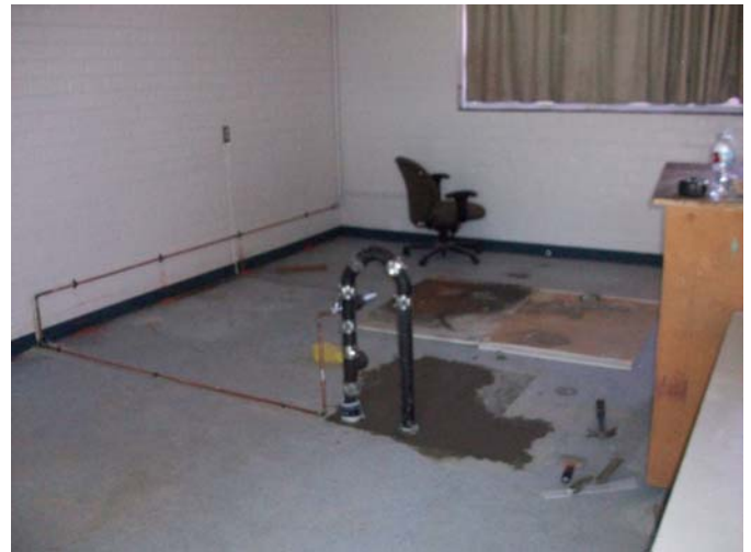
2. Building B- Rough-in plumbing in classroom 16 complete.
