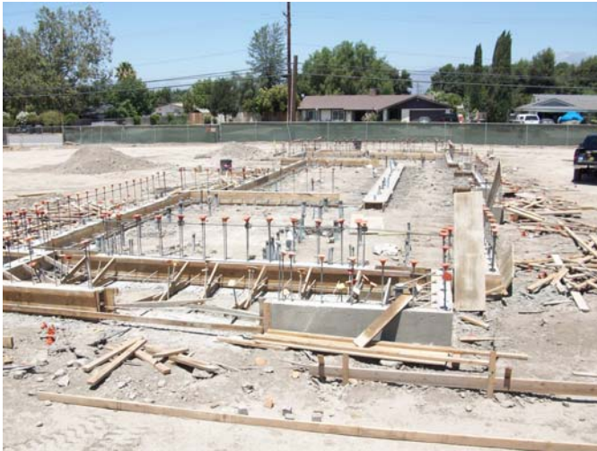
1. Building A- Removing form work.
