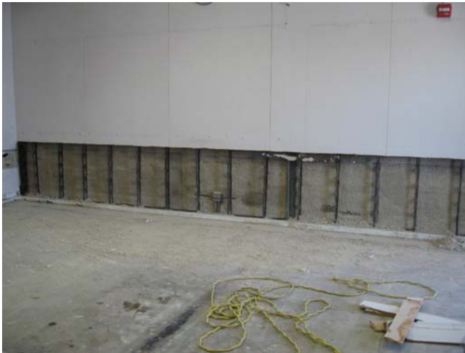
1. Building A- Open wall ready to receive casework backing.
