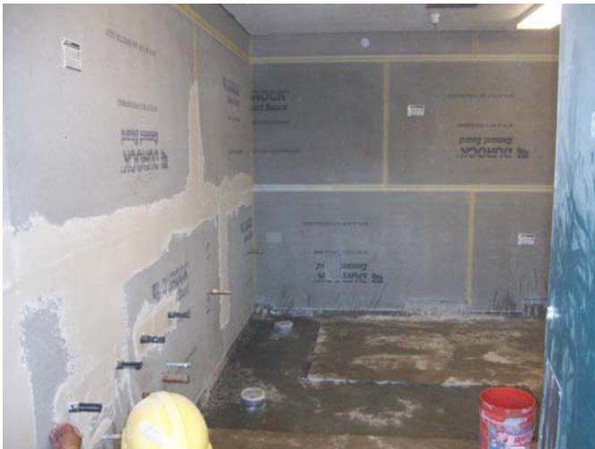
3. New backer board at restroom complete.
