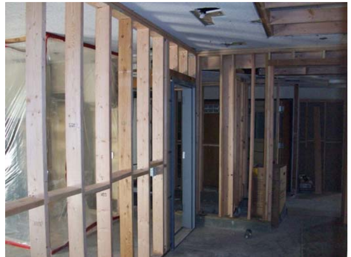
4. New wood walls and HM frame complete.
