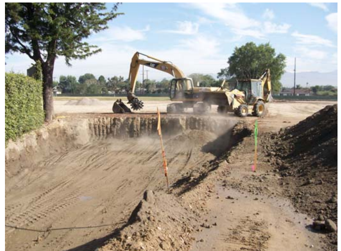
4. Over-excavation for stair bleachers. .
