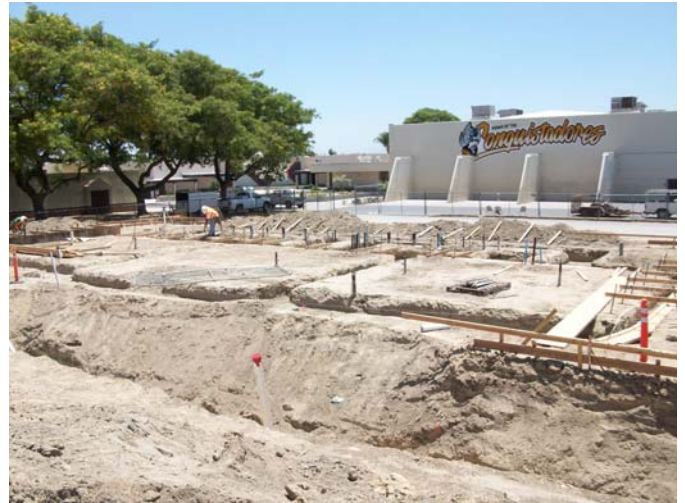
2. Building B- Setting form work has begun.
