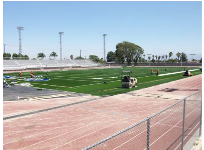
2. Chino HS- Installing new field turf material
