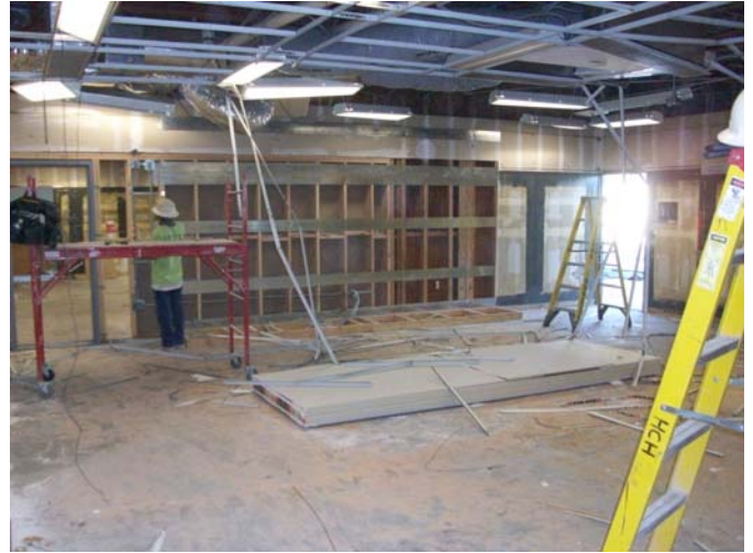
2. Installation of casework backing and drywall on-going.
