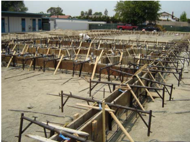
1. Construction of perimeter stemwall formwork (looking north).
