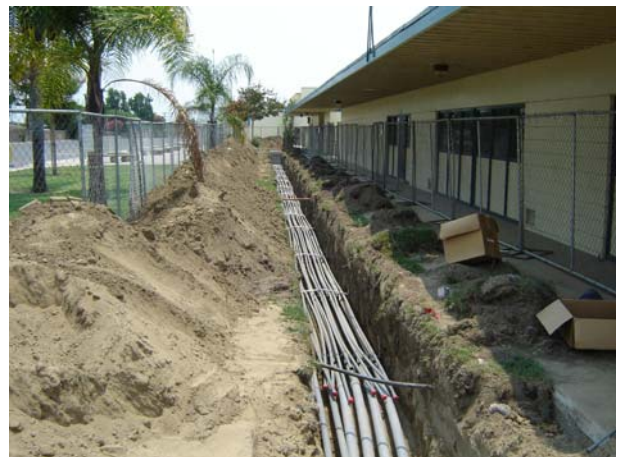
2. Trenching/conduit from Administration to New Classroom.
