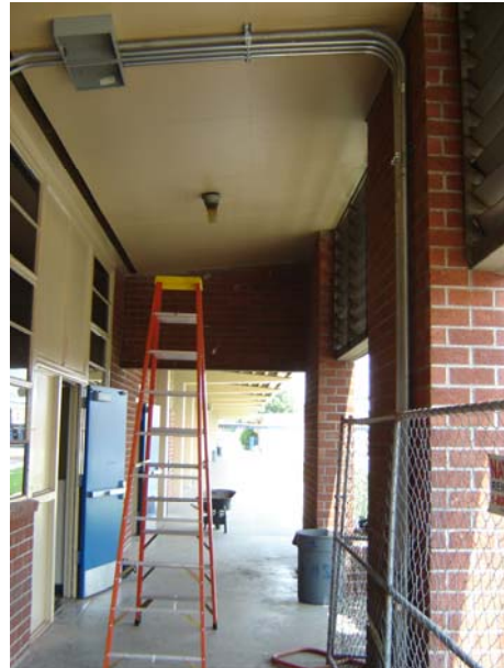
4. Electrical conduit for Relocatable Restroom.
