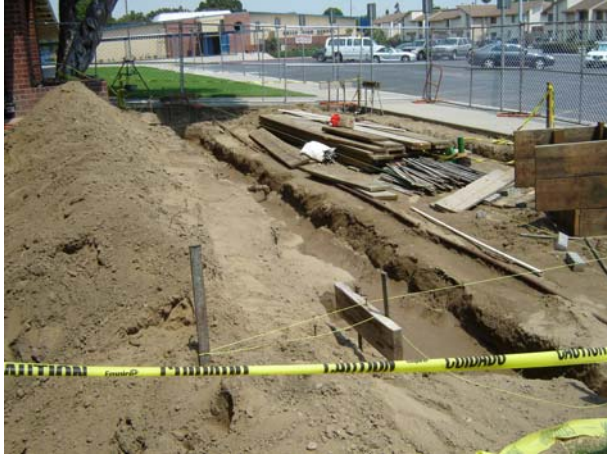
1. Excavation for footing at Relocatable Restroom.
