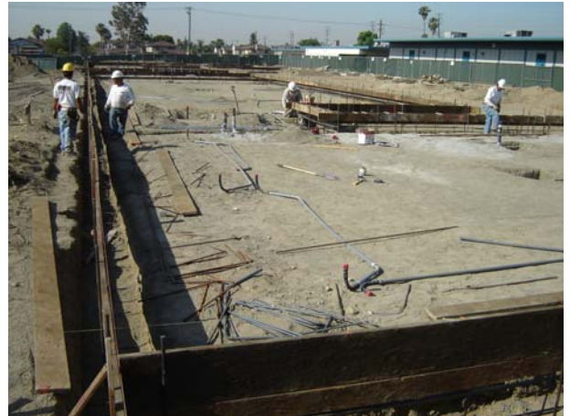
2. Construction of perimeter stemwall formwork (looking south).
