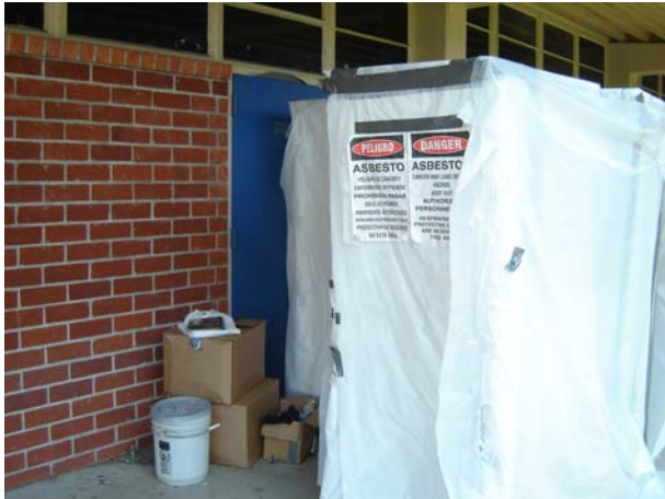
3. Asbestos abatement of classroom floor tile.
