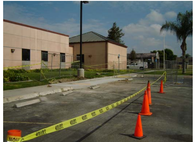
4. Installed new concrete ADA ramp.
