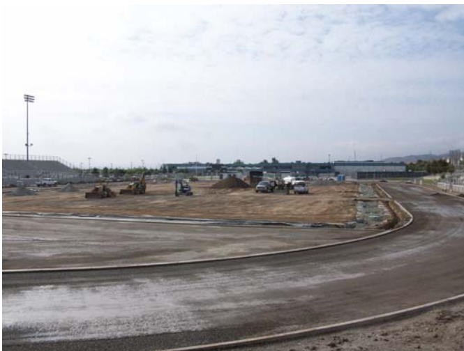
3. Chino Hills HS- Installing base at the track, ready to be paved.
