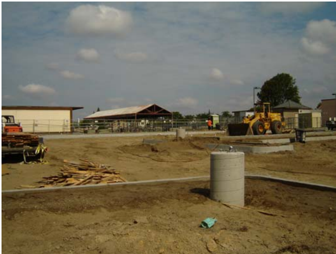
3. Installed concrete curb and light pole stands.
