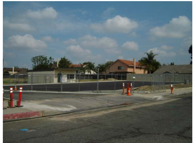
4. Installed AC paving at the staff's parking lot.
