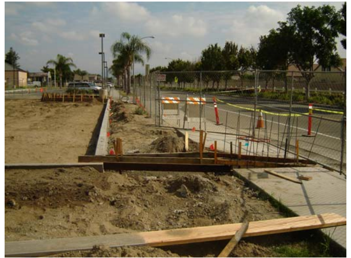
2. Installed form work for concrete culvert and irrigation lines.
