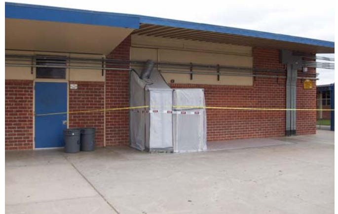
2. Counseling Building- Removal of VAT material complete.
