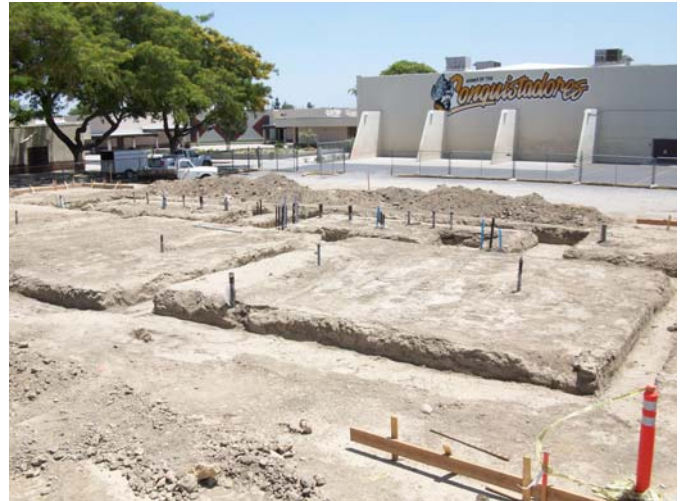
2. Building B- Building footings in-progress, ready to set form work.
