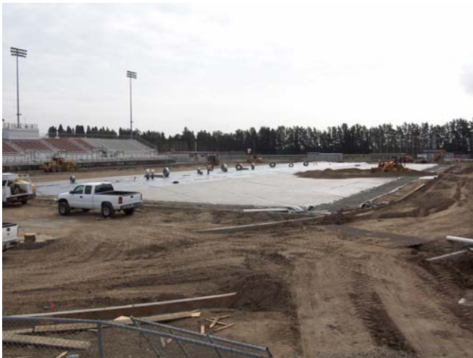
1. Ayala HS- Installing permeable system on the field.
