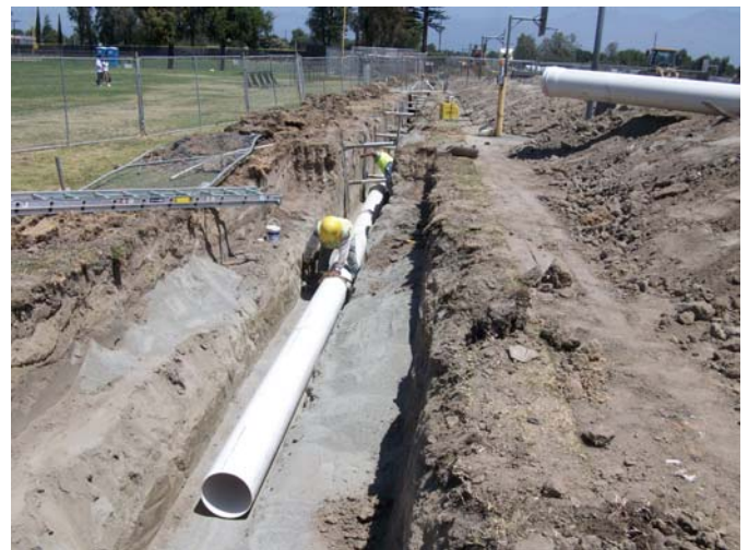
4. Installation of storm drain SDR-35 pipe on-going.
