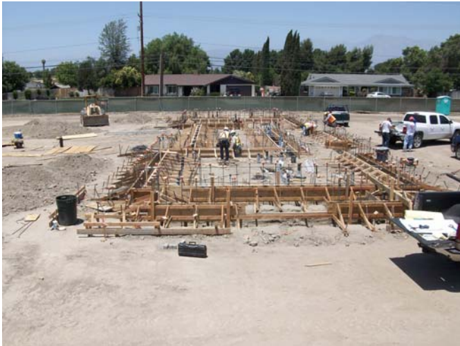
1. Building A- Form work and rebar complete, rough elect. on-going.
