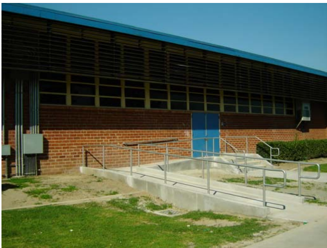
3. New ADA concrete ramp with hand rails.
