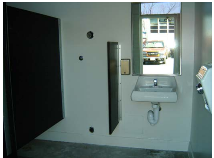
4. New plumbing fixtures, partition walls and toilet accessories.
