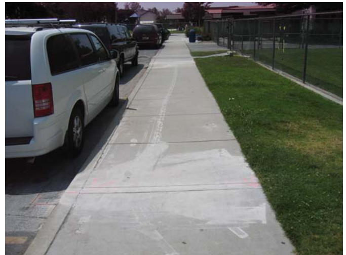
4. Saw cut for new ramps is complete.
