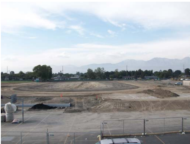
3. Over-excavation and re-compaction at the field on-going.
