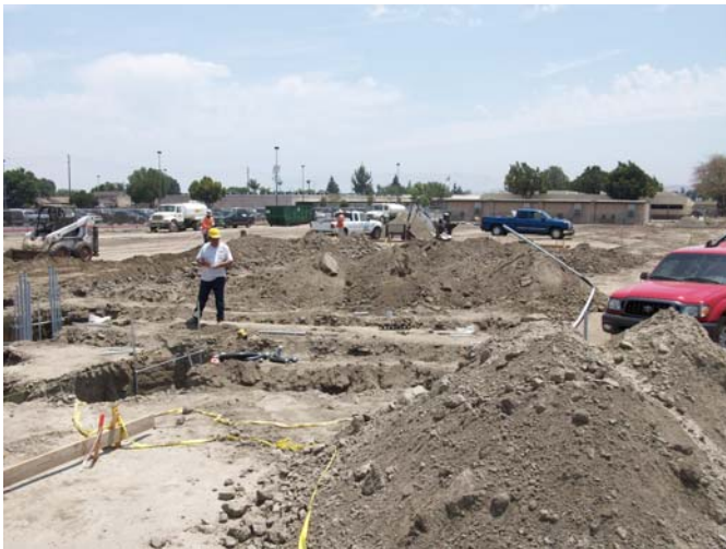
1. Building A- New underground electrical and plumbing on-going.
