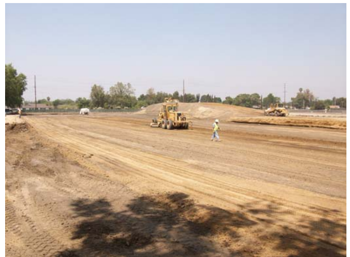
4. Removal of existing curb, gutter and storm drain complete.
