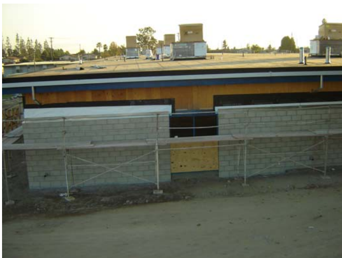
3. Completed CMU veneer and scaffolding for exterior plaster.
