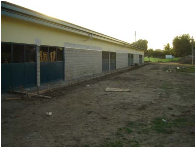
1. CMU block veneer and painted plaster.
