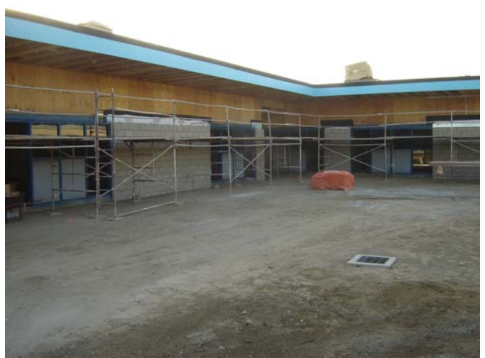
4. Completed hollow metal door/window frames.
