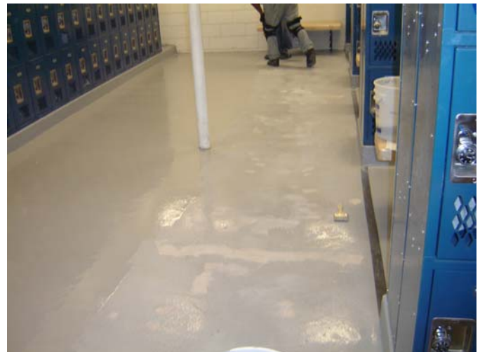
4. Epoxy coating in Locker Rooms.
