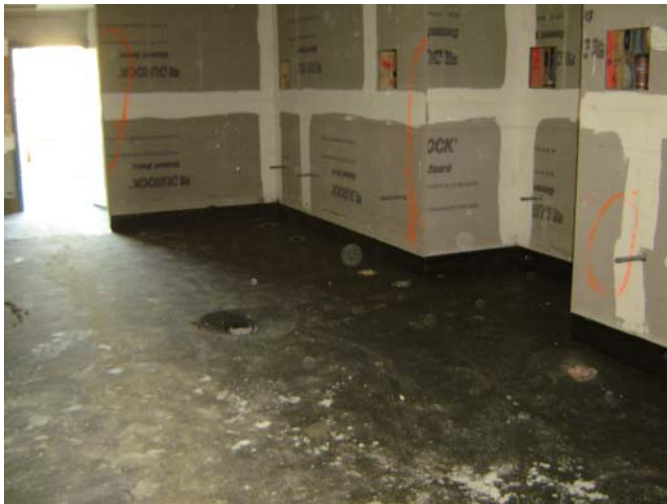
1. Mortar bed for floor tile and cementitious wall board in Restroom.
