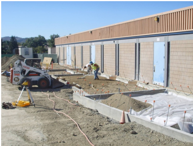
3. Preparing for slab-on-grade pour.
