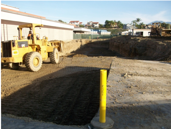
1. Backfilling the building pad.
