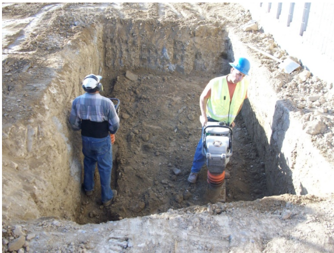
3. Soil compaction of slots.
