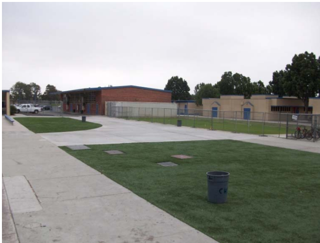
3. New concrete fire lane and hydrosed planter complete.
