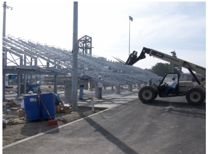
2. Bleacher installation in progress.
