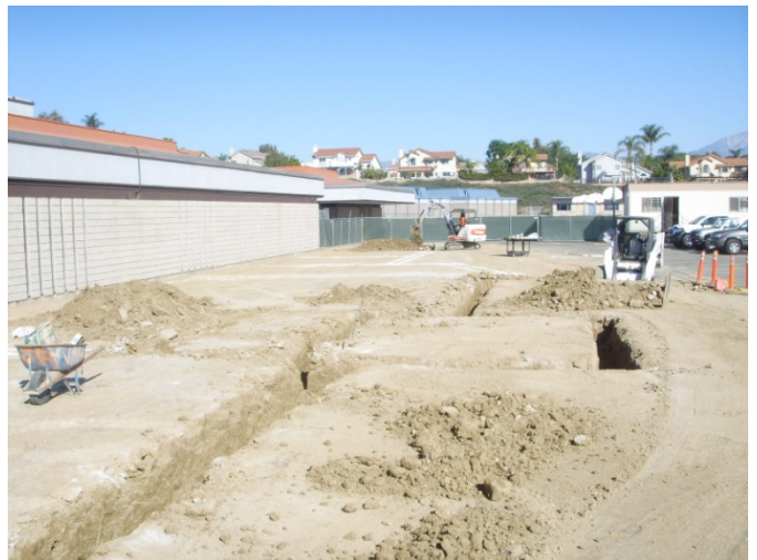
4. Footing excavation has begun.
