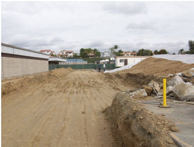
3. Demolition and overexcavation.
