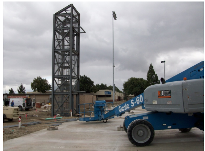
4. Structural Steel for elevator tower.
