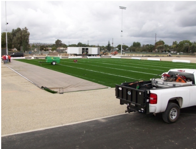
1. Field Turf installation in progress.
