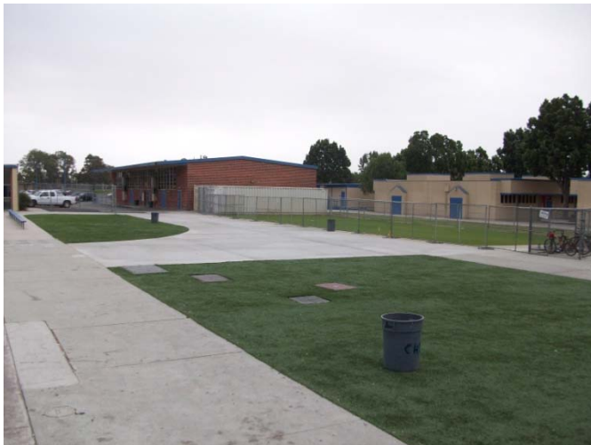
3. New concrete fire lane and hydrosed planter complete.
