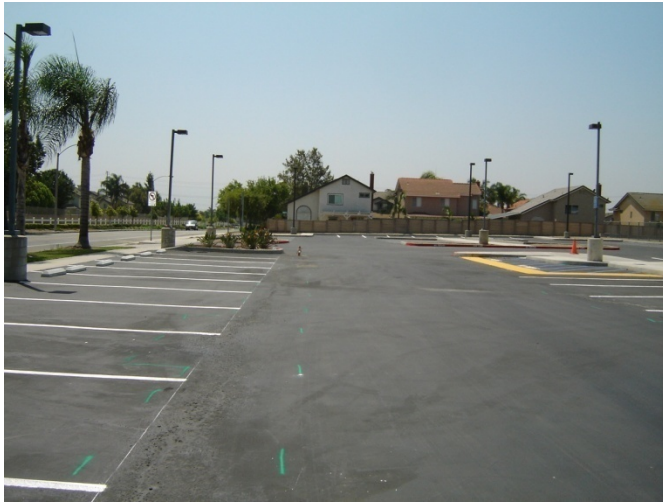
1. New asphalt paving and wheel stops complete.
