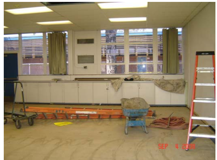
2. Completed floor removal and electrical rough-in.
