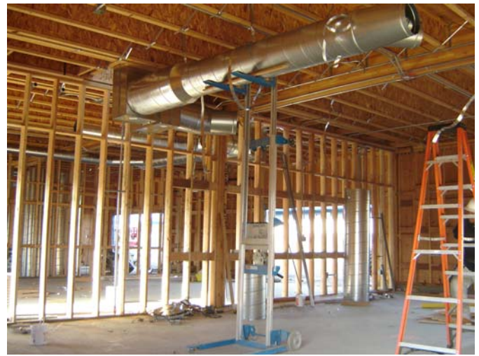
4. Interior wood framing and ductwork installation.
