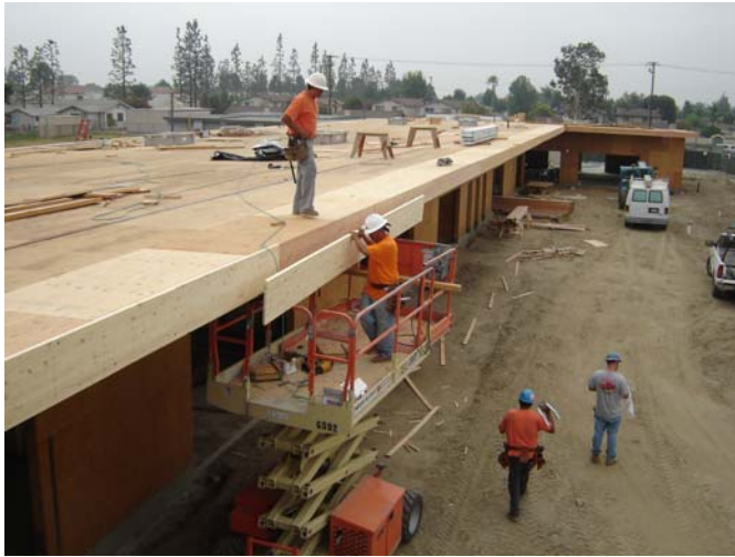
1. Installation of fascia board.
