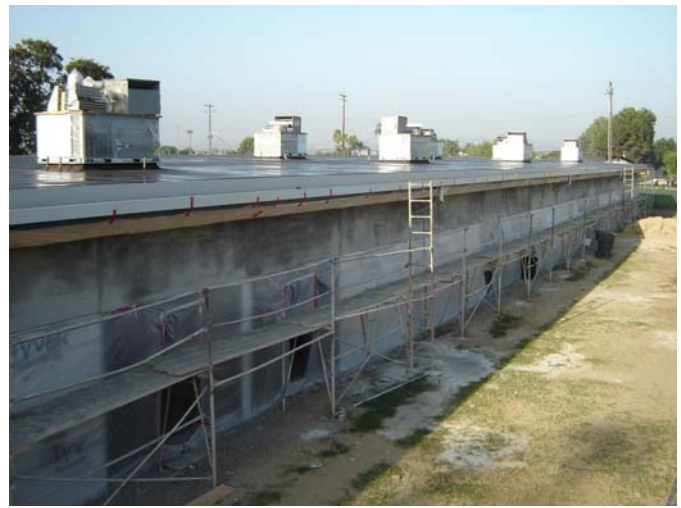
2. Completed brown coat of plaster.
