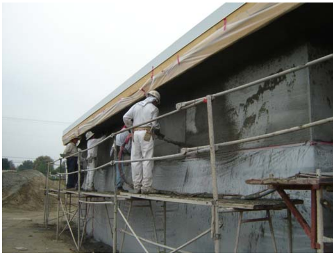
1. Applying brown coat of plaster.
