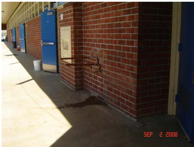
1. New doors and plumbing rough-in for drinking fountains.
