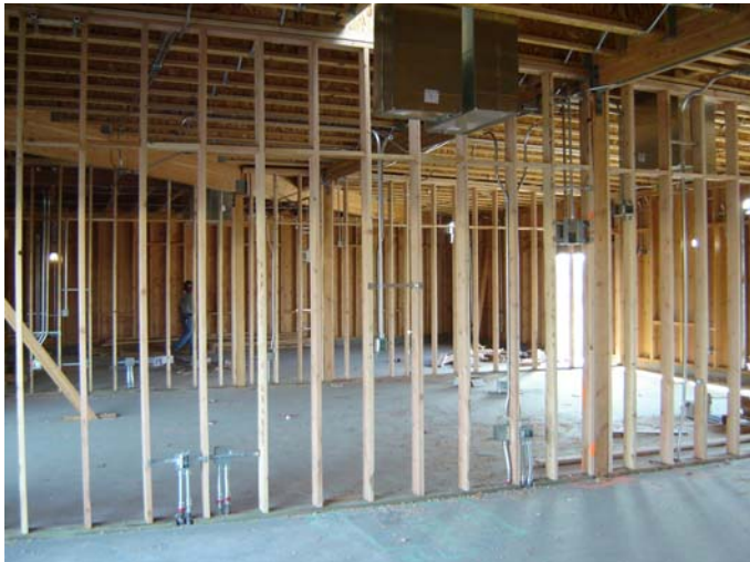
3. Interior wood framing and electrical rough-in.
