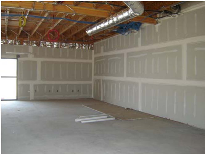
3. Drywall taped interior walls.
