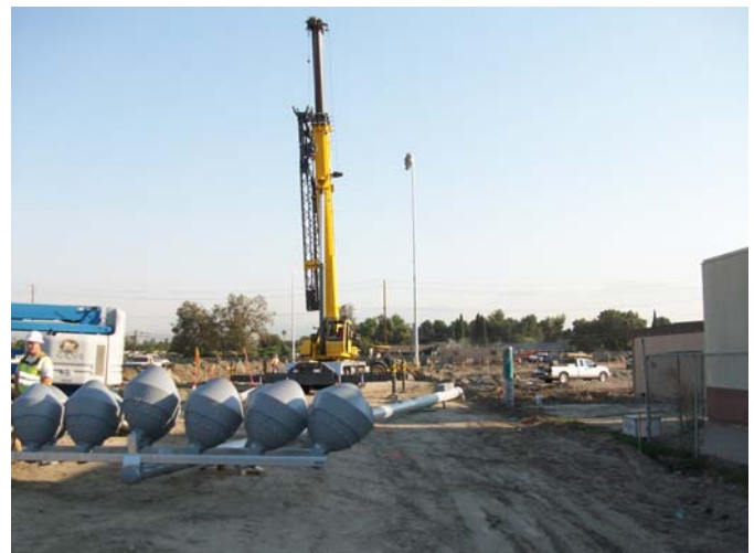
4. Erecting new light poles.
