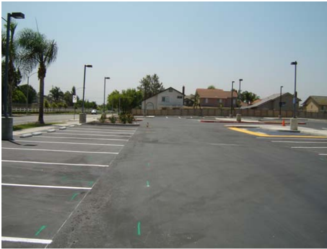
1. New asphalt paving and wheel stops complete.
